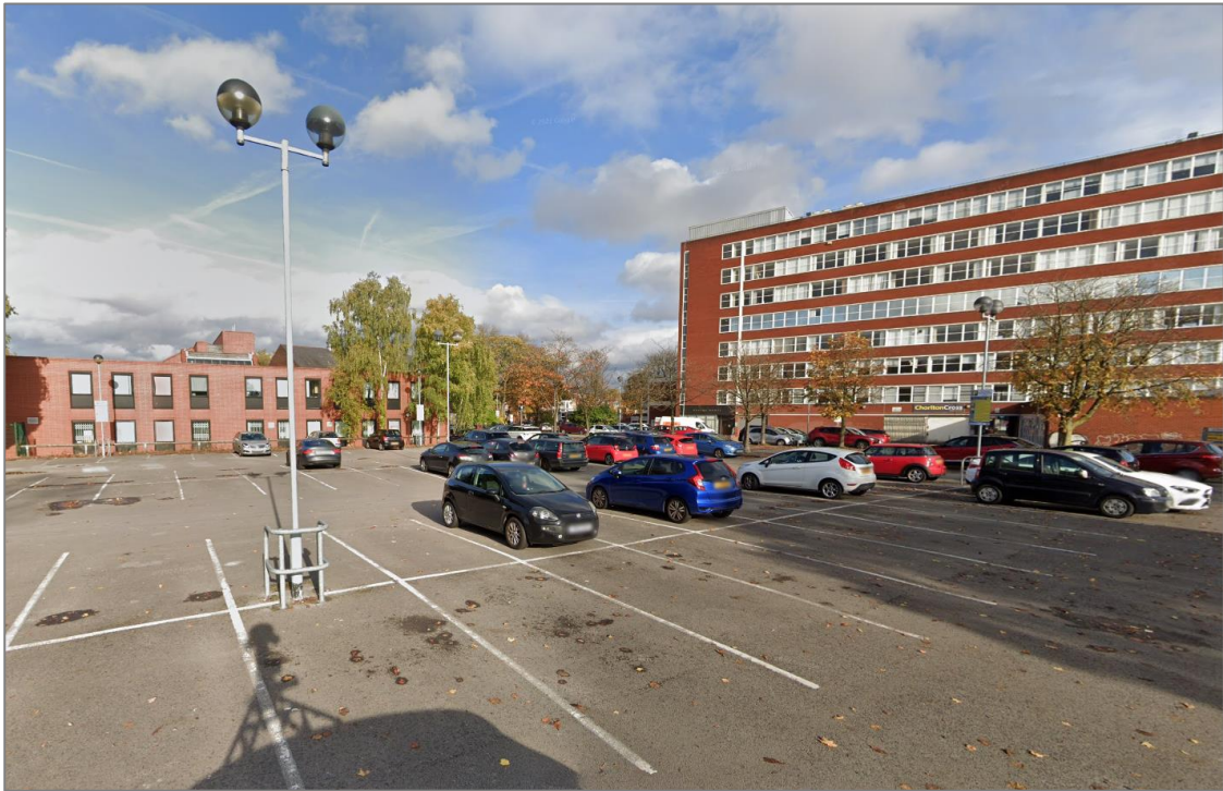
Figure 2. Existing site lighting
