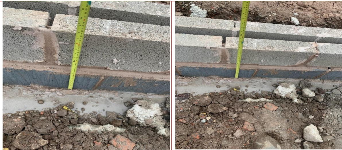
Sub Floor Void – Plot 201
