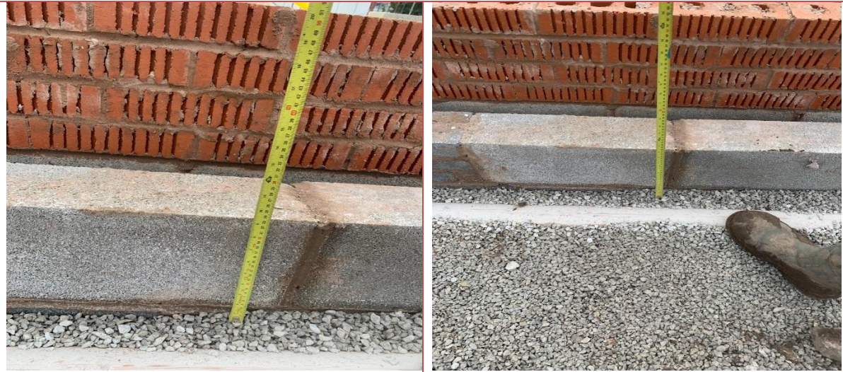
Sub Floor Void – Plot 200
