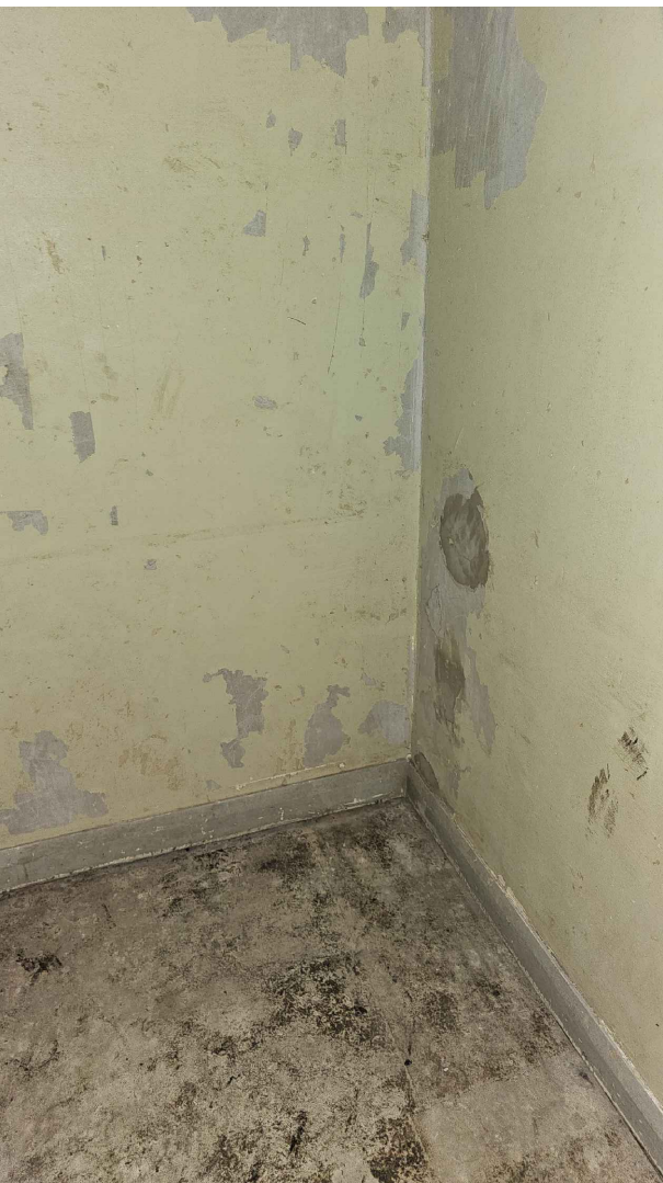
WALLS 9-12 MODERN LINING
