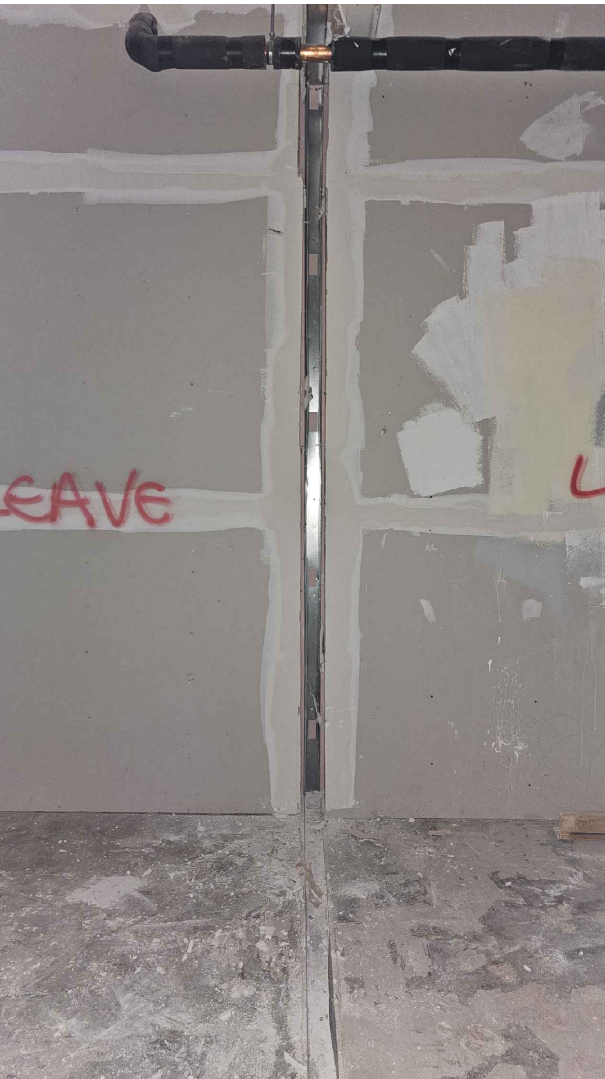
WALL 6 MODERN LINING PLASTERBOARD.
