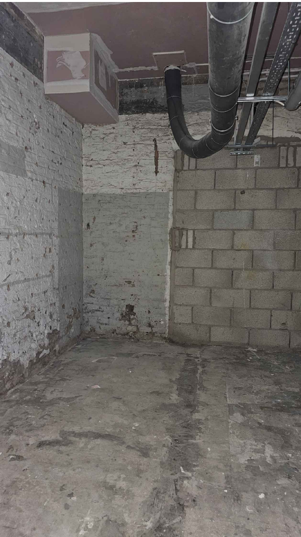
WALL 7 ORIGINAL FABRIC AND MODERN BLOCKWORK WALL 8 ORIGINAL FABRIC
