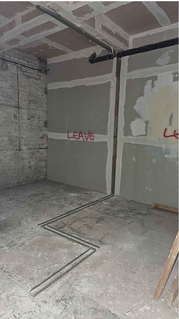
WALL 6 MODERN LINING PLASTERBOARD. WALL 7 ORIGINAL FABRIC
