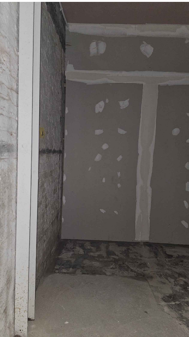
WALL 2 MODERN LINING PLASTERBOARD WALL 3 ORIGINAL FABRIC
