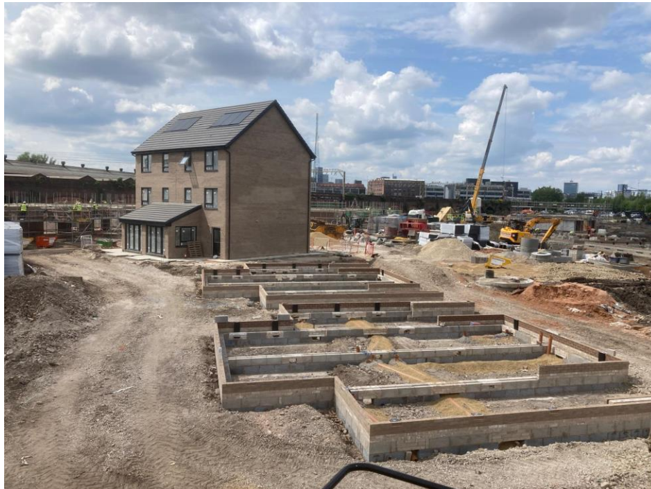
Plate 2 – Subfloor Void Space and Vents Prior to Block and Beam
