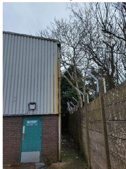
Photo 6: T63 – T67, looking west
