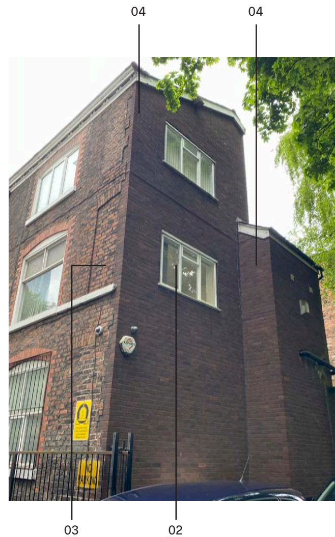
Mid-late century facade along demolition line of former terraced housing on Longworth Street
