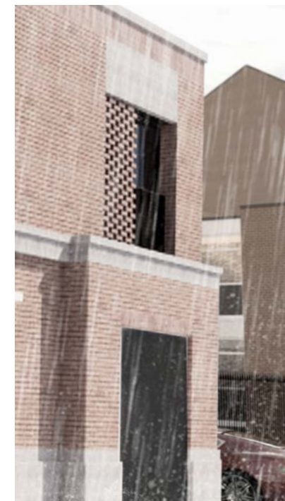
Brickwork articulation and wetcast concrete window detailing
