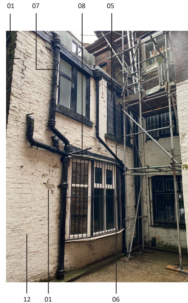
19th century lean to outrigger built to house the existing staircase to No. 8. Split pitched roof and dormer
