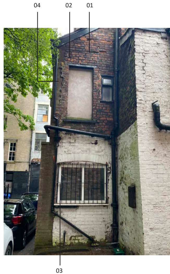
Former rear elevation of demolished Longworth Street terraced houses
