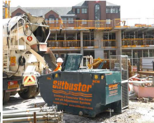
ROADSIDE CONCRETE WASHOUT (RCW)
