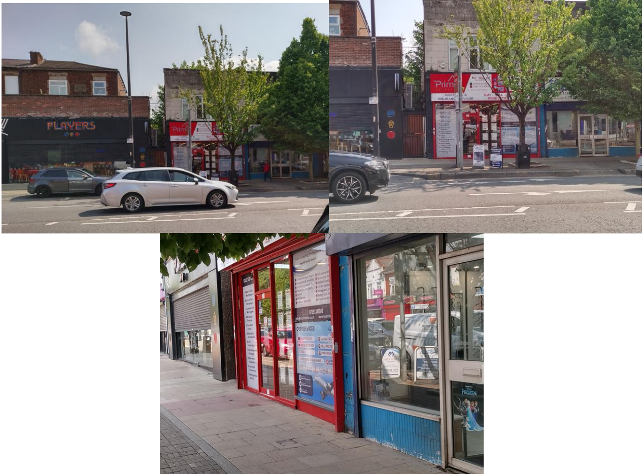
Fig.1 – Views of the frontage to 58A Bury Old Road
