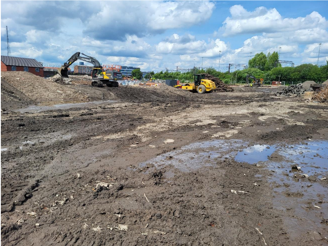
Pic 3 – Remediation works being undertaken
