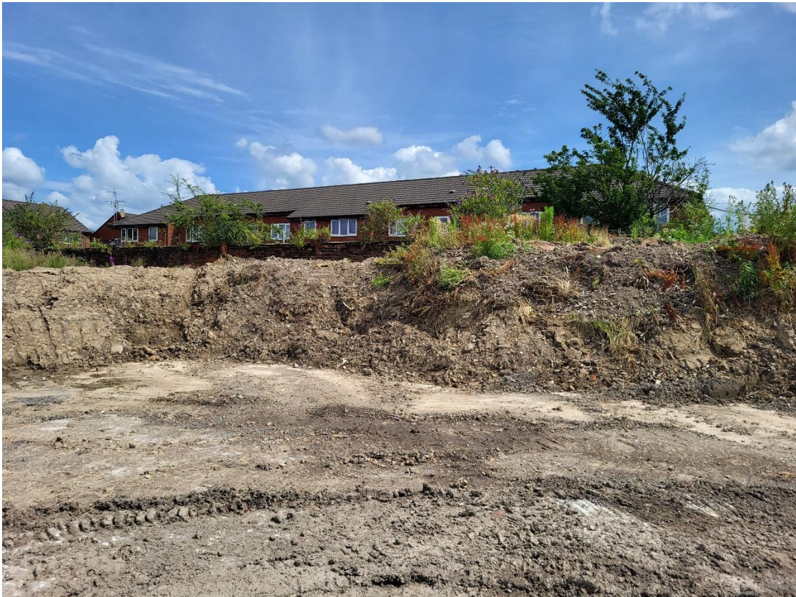
Pic 4 – Spoil stockpiles along eastern boundary
