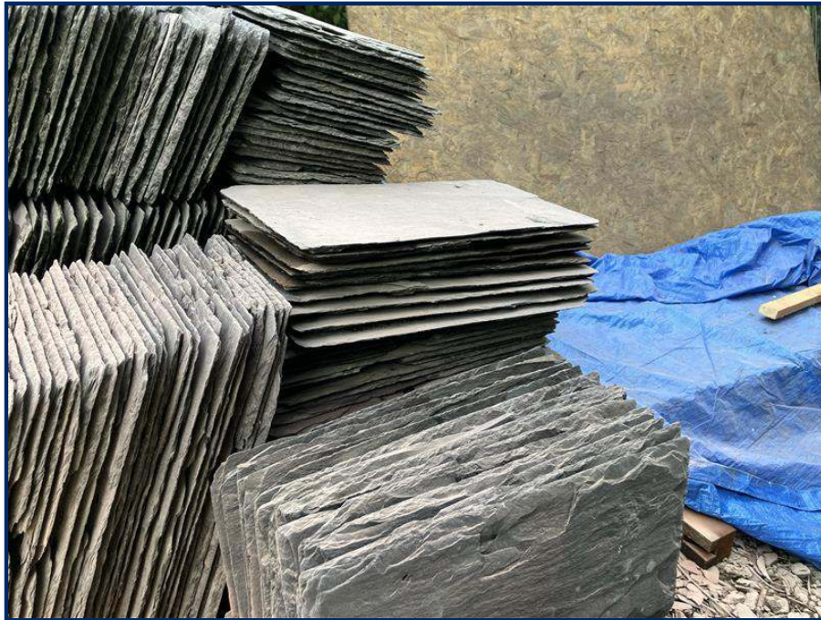
Photo [11] - Proposed Natural Welsh Slate as per the existing
