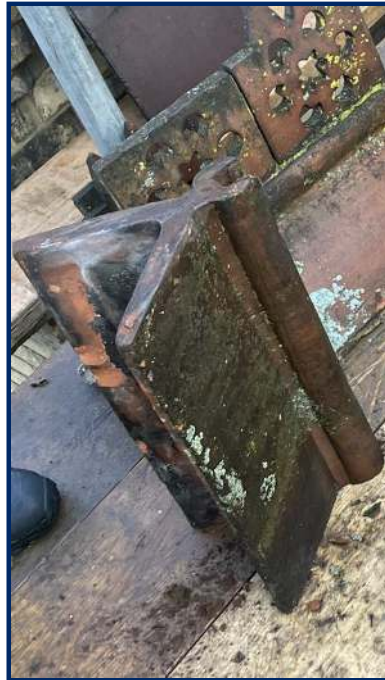
Photo [5] - Existing Ridge Tile
