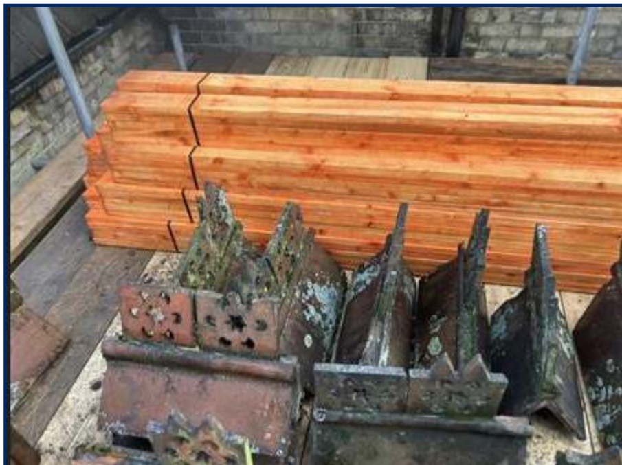
Photo [6] - Existing Ridge Tiles and Inserts
