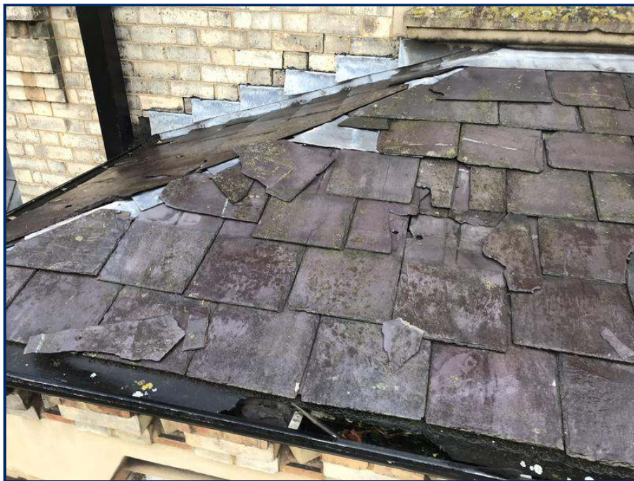
Photo [1] - Existing Slates
