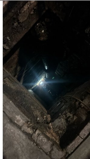
Manhole / Access Point: MH1 Internal
