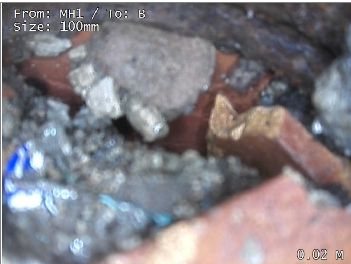
Collapsed drain/sewer 100%
