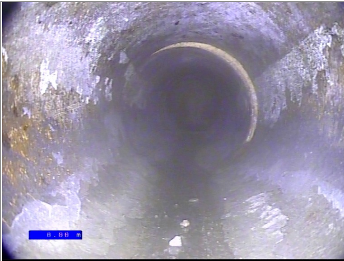
Start node type, manhole, reference MH1
