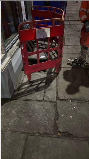
Manhole / Access Point: MH1 Location
