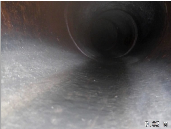
Start node type, manhole, reference MH1
