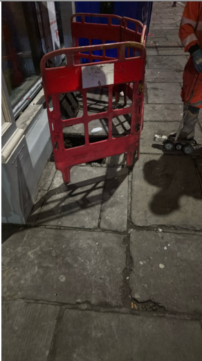
Manhole / Access Point: MH1 Location
