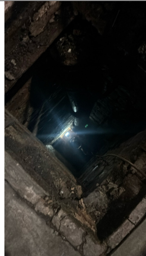
Manhole / Access Point: MH1 Internal
