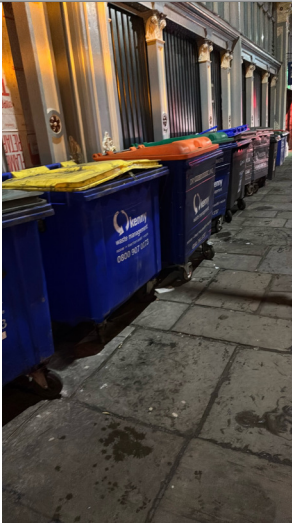
Other Site Photos: No MH underneath bins
