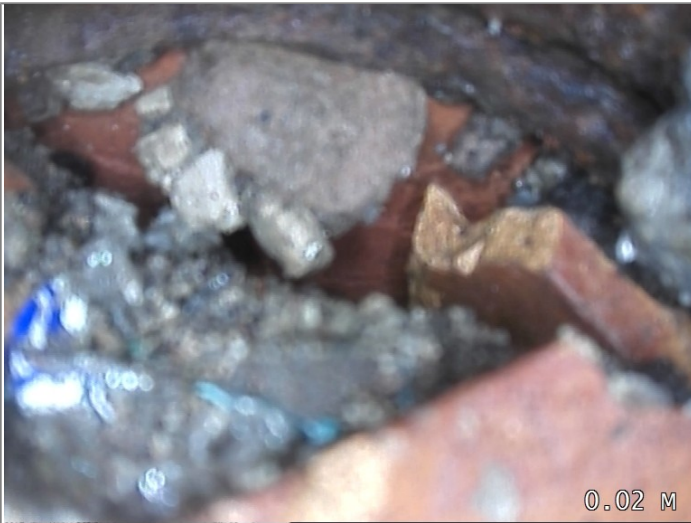
Start node type, manhole, reference MH1
