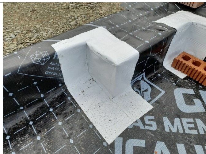
Evidence of sealing of membrane
