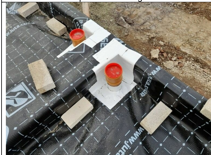
Evidence of sealing of service entries
