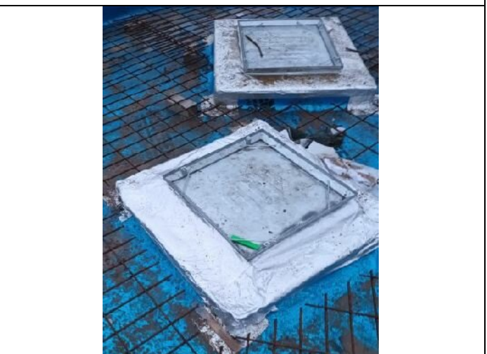
Sealing of internal manhole covers
