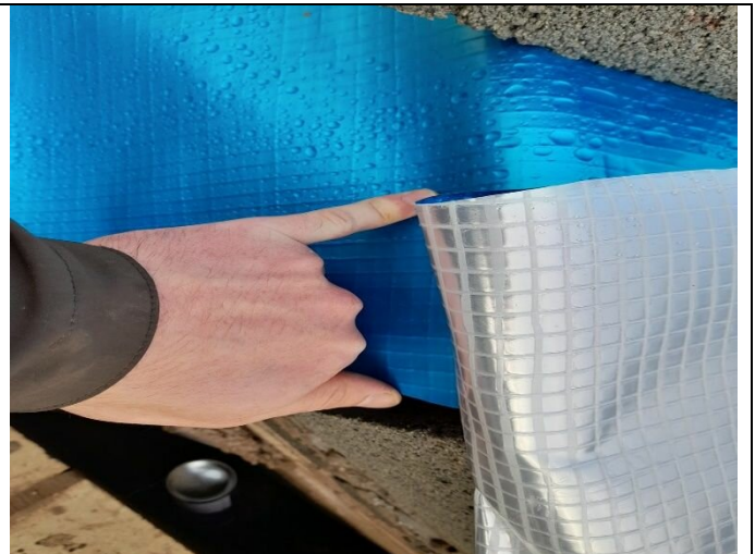
Example of overlapping of gas membrane in the apartment building.
