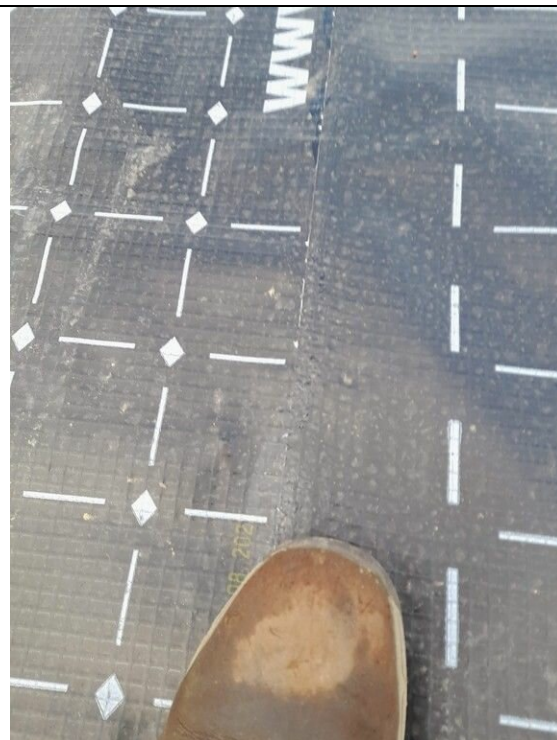
Evidence of welding of the membrane
