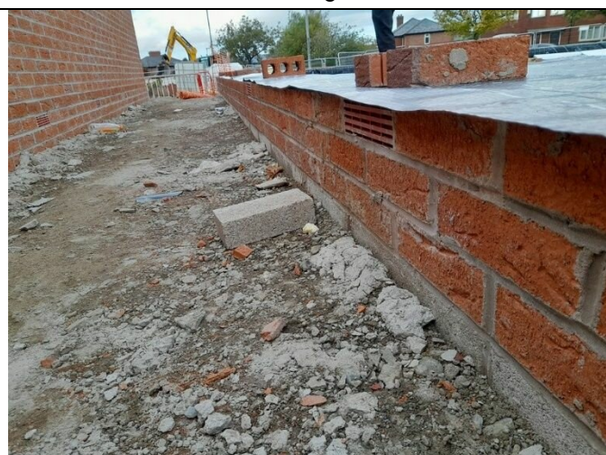
Evidence of vented air bricks to the apartment building
