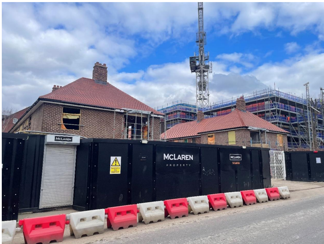
Figures 8: Looking east from the eastern end of the Site on Oxford Place during construction in May 2025, illustrating the height of the new build element to the far right.
