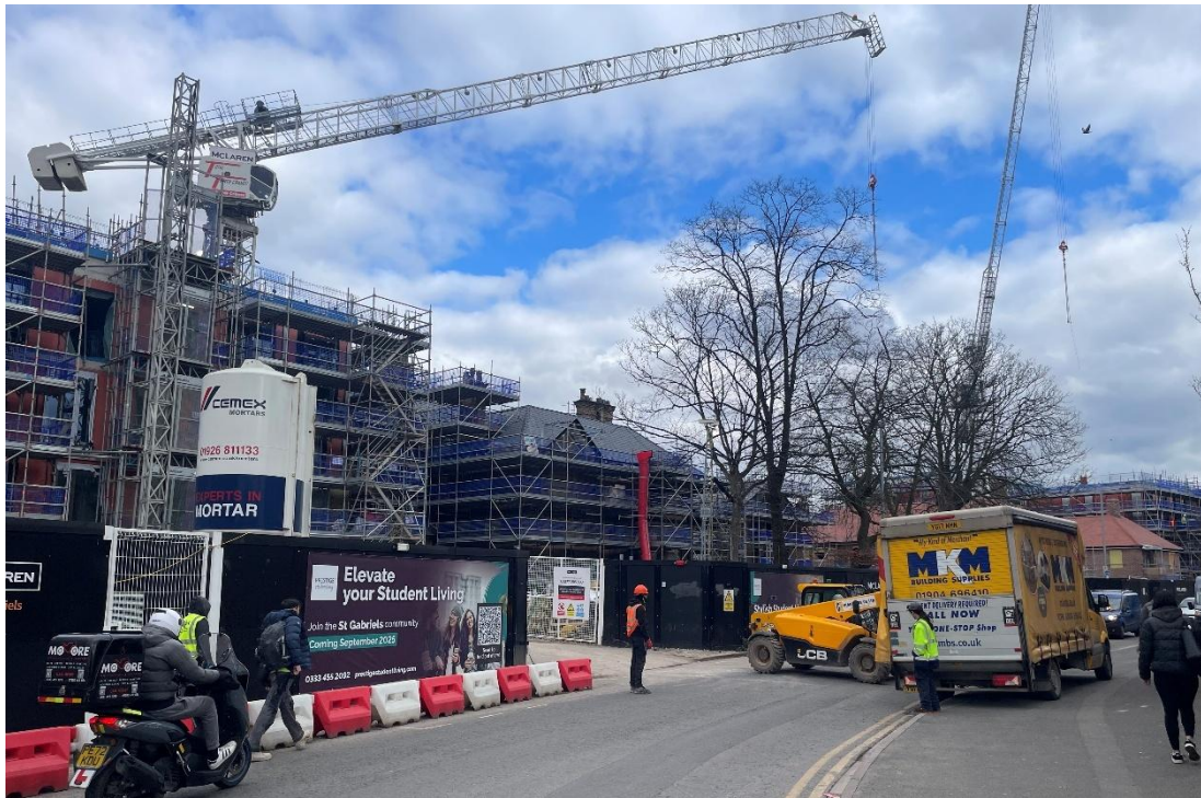
Figures 7: Looking east from the western end of the Site on Oxford Place during construction in May 2025, illustrating the height of the new build element to the far left.
