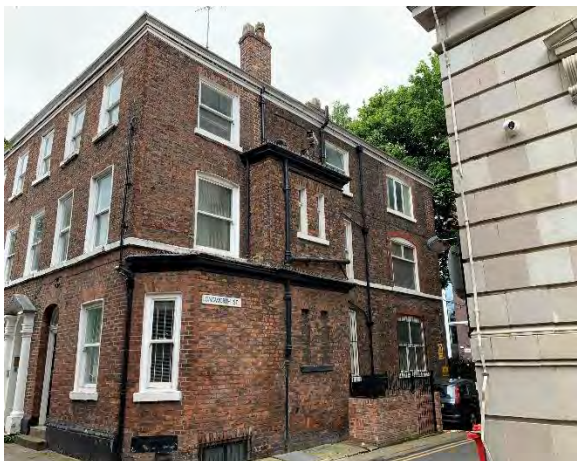
Figure 2.3: Longworth Street and access to basement on east of No. 8a.
