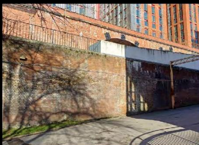
Level change between Altrincham Street and the rest of the site below - from the service road
