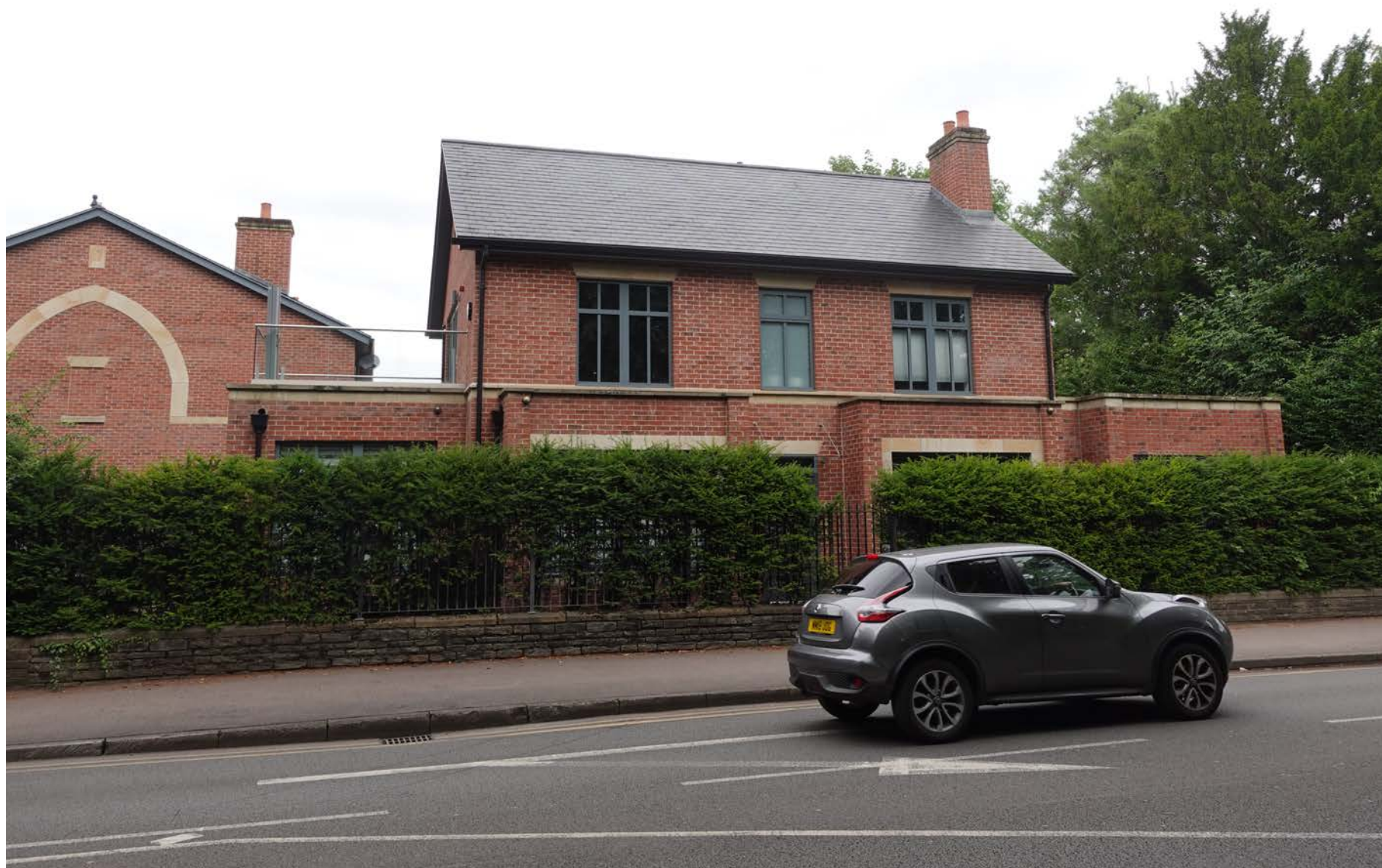
Image: Views of 72 Bloomesbury Avenue. Wilmslow Road Rear Elevation (Above) / Bloomesbury Avenue Front Elevation (Right)
