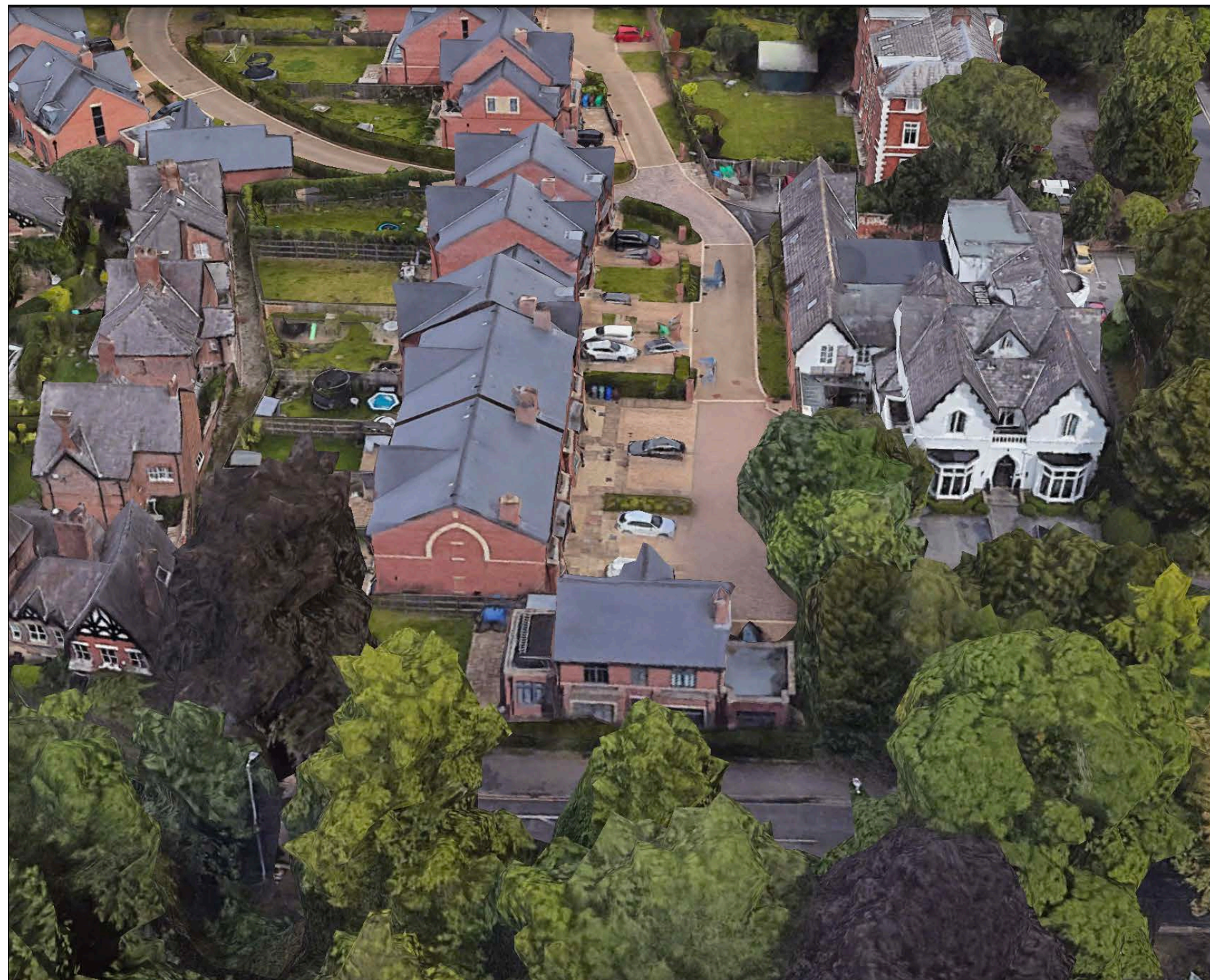
Image: Aerial View of 72 Bloomesbury Avenue showing flat roof to both sides of the property creating an elongated base out of character with the context.
