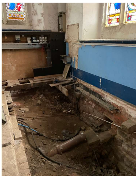
Existing foul drainage beneath floors
