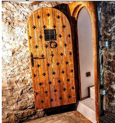
Example of open grate to an historic door
