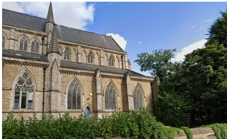
West facing elevation with small side entrance
