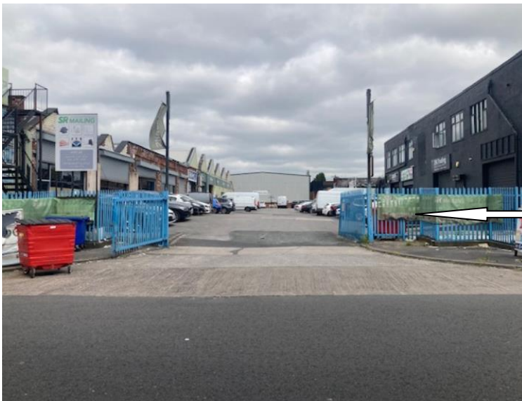
View of the access into the development and car park from Derby Street. The position of the proposed building is indicated by the arrow.
