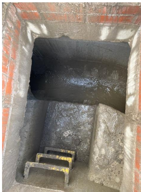
Photographs showing the construction of adoptable 1800mm diameter SW highway drain manholes in accordance with approved Manchester Highways standard construction details, as approved under the Section 38 agreement. (Left: MH S1; Right: MH S2).
