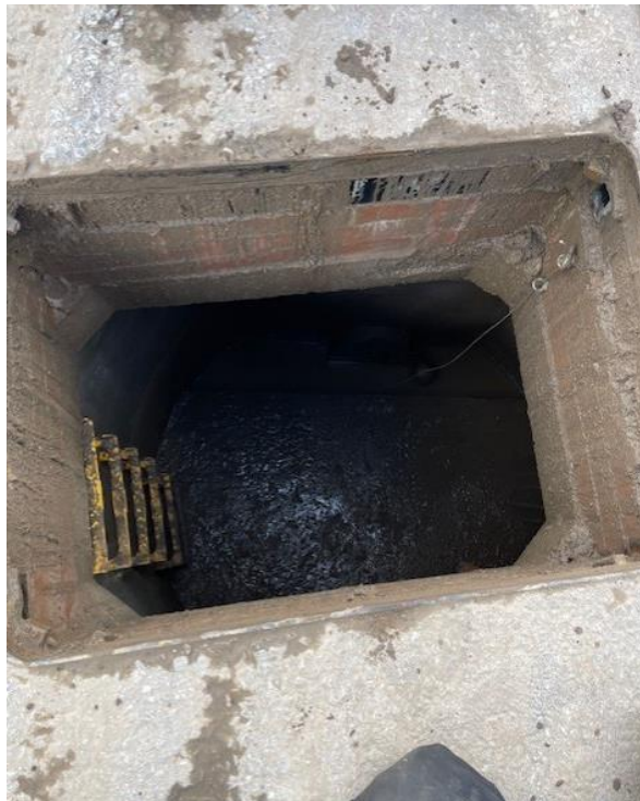
Photographs showing the construction of adoptable SW highway drain flow control manhole (S3) in accordance with approved standard detail.
