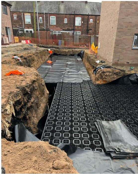
Photographs showing the private attenuation tank has been constructed in accordance with approved standard details and to the correct size, depth and invert level with suitable cover.
