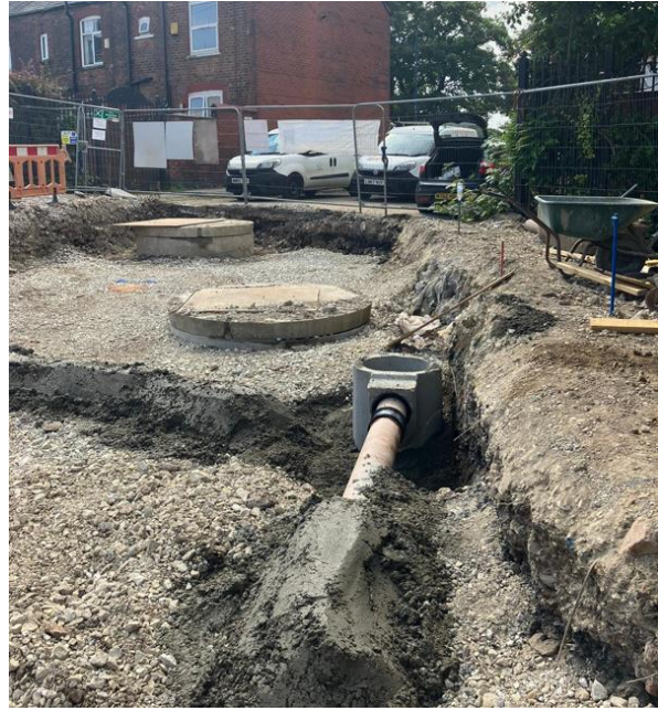
Photographs showing the construction of adoptable SW highway gullies in accordance with Manchester Highways standard details, as approved under the Section 38 agreement.
