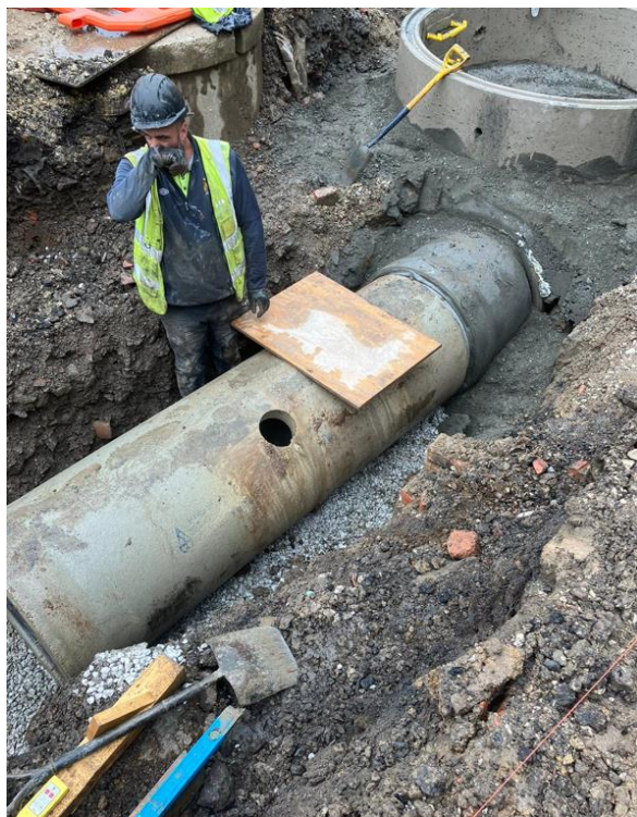
Photographs showing the construction of adoptable 600mm diameter SW highway drain from MH S2 to S3 in accordance with Manchester Highways standard details, as approved under the Section 38 agreement.
