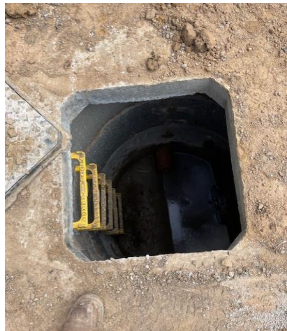
Photographs showing the construction of the private flow control chamber S4 have been constructed in accordance with DCG guidance and Hydro International specialist design drawings.
