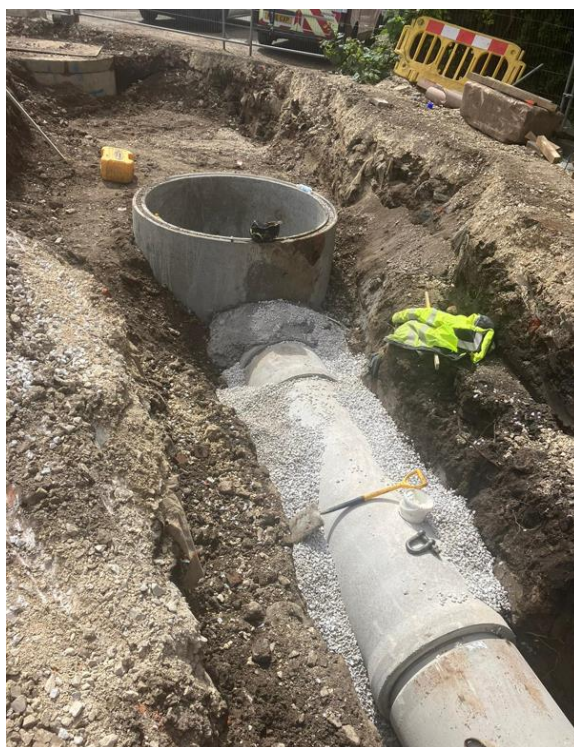
Photographs showing the construction of adoptable 600mm diameter SW highway drain from MH S2 to S3 in accordance with Manchester Highways standard details, as approved under the Section 38 agreement.
