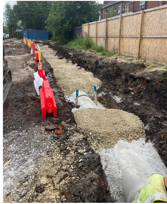
Photographs showing the construction of adoptable SW highway gullies in accordance with Manchester Highways standard details, as approved under the Section 38 agreement.
