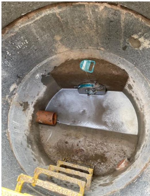
Photographs showing the construction of the private flow control chamber S4 have been constructed in accordance with DCG guidance and Hydro International specialist design drawings.
