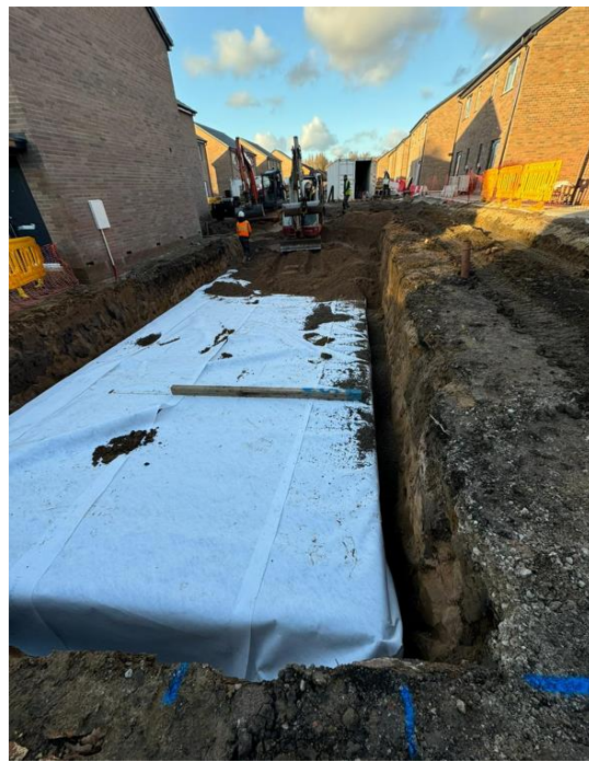
Photographs showing the private attenuation tank has been constructed in accordance with approved standard details and to the correct size, depth and invert level with suitable cover.
