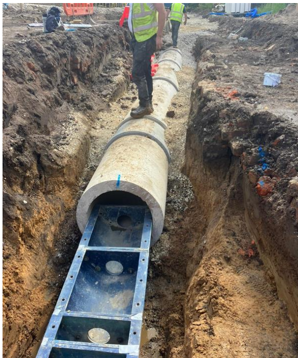
Photographs showing the construction of adoptable SW highway gullies in accordance with Manchester Highways standard details, as approved under the Section 38 agreement.
