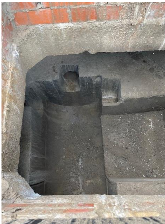
Photographs showing the construction of adoptable 1800mm diameter SW highway drain manholes in accordance with approved Manchester Highways standard construction details, as approved under the Section 38 agreement. (Left: MH S1; Right: MH S2).
