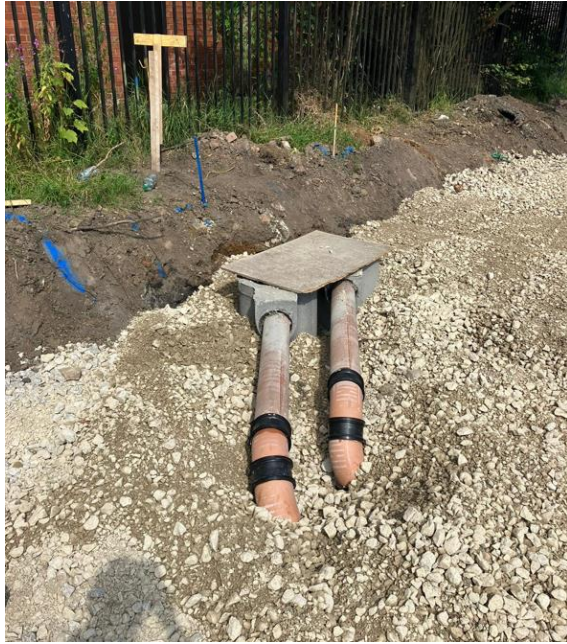
Photographs showing the construction of adoptable SW highway gullies in accordance with Manchester Highways standard details, as approved under the Section 38 agreement.
