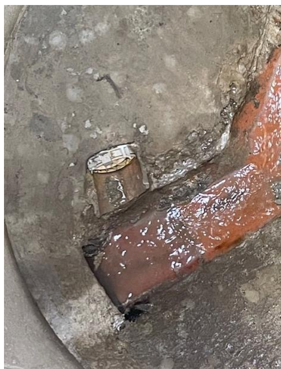
Photographs showing the construction of new incoming connections from new drainage systems into the existing, United Utilities combined manhole C7 in accordance with United Utilities and DCG approved requirements as agreed in the Section 106 application.
