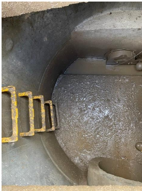
Photographs showing the construction of adoptable SW highway drain flow control manhole (S3) in accordance with approved standard detail.
