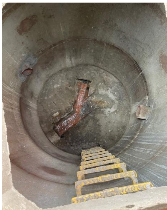
Photographs showing the construction of new incoming connections from new drainage systems into the existing, United Utilities combined manhole C7 in accordance with United Utilities and DCG approved requirements as agreed in the Section 106 application.
