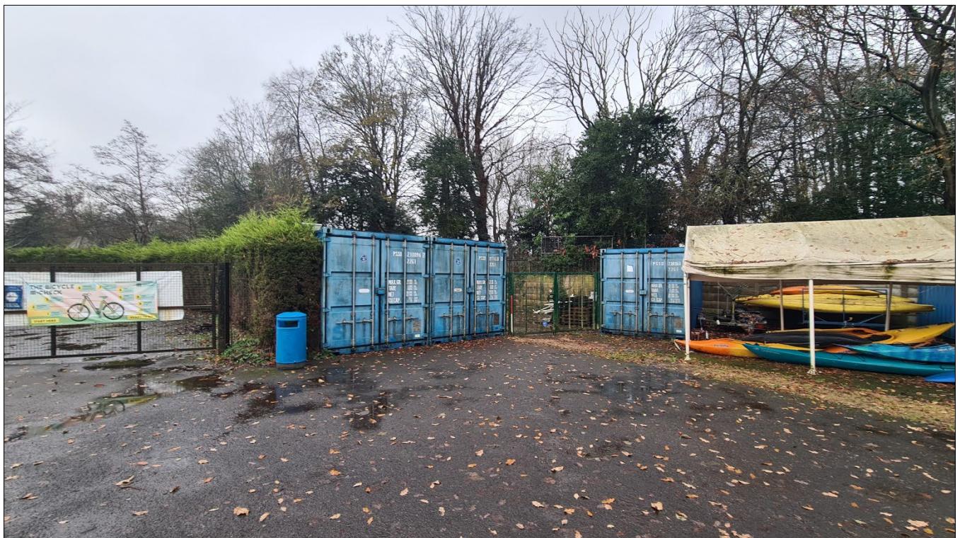
Photograph 2) View of the southern section of the Site, facing southwest
