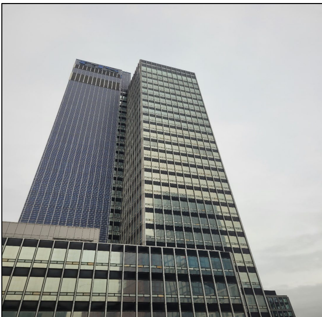
Photograph 3 The CIS tower taken from the east
