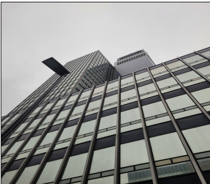
Photograph 6 The predominantly glazed exterior of the tower and podium building
