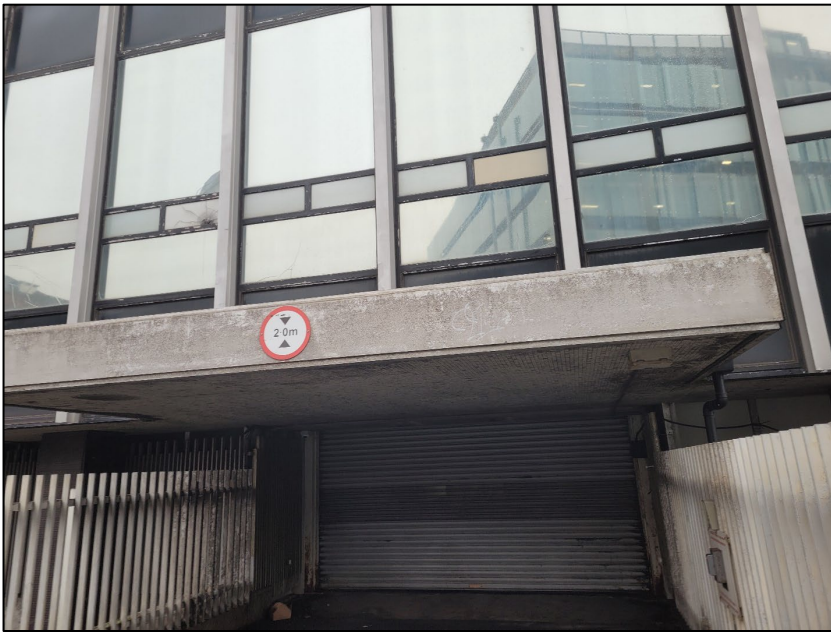
Photograph 7 Example of glazing, steel mullions and concrete block
