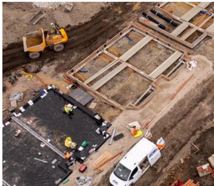
Membranes installed on plots 139-140 with JCW on site installing gas membranes
