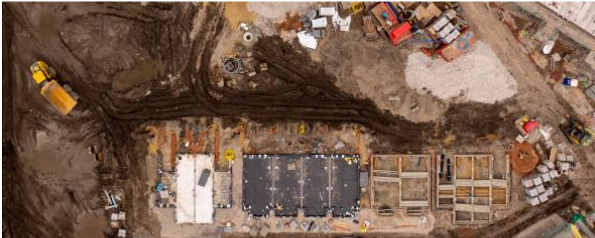
Membranes installed on plots 143 - 146
