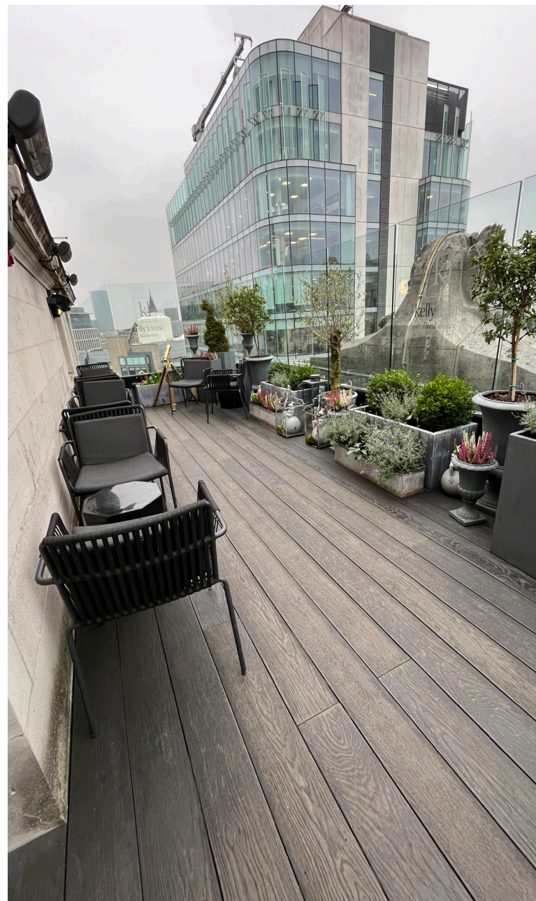
Image: External decking to 100 King Street.
