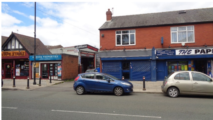
Adjoining Properties to Application Property.
