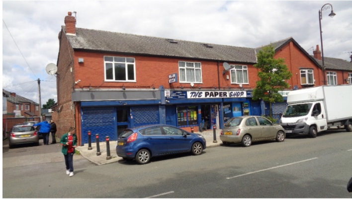
Front Elevation to Application Property.
