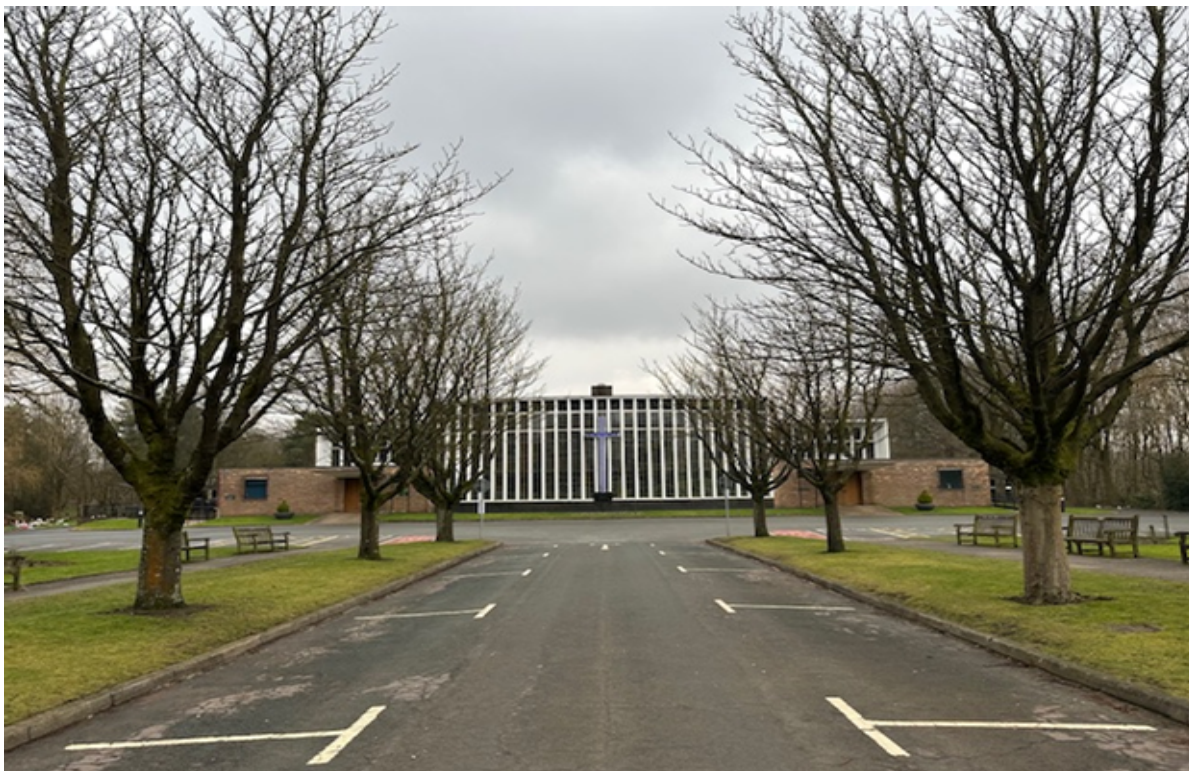
View southwest of principal elevation of Blackley Crematorium from the tree lined avenue (Rose Walk) due NE.
