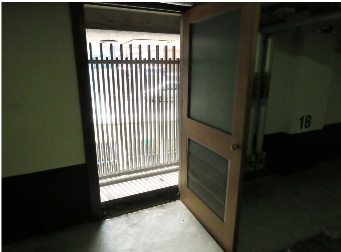
00m-05 The escape doors on the south elevation, showing the doors and external railings.
