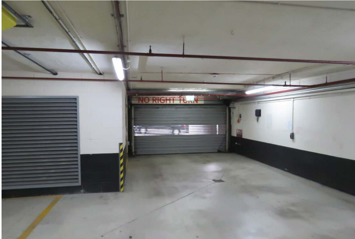
00m-04 Looking east towards the vehicle entrance from Hanover Street.
