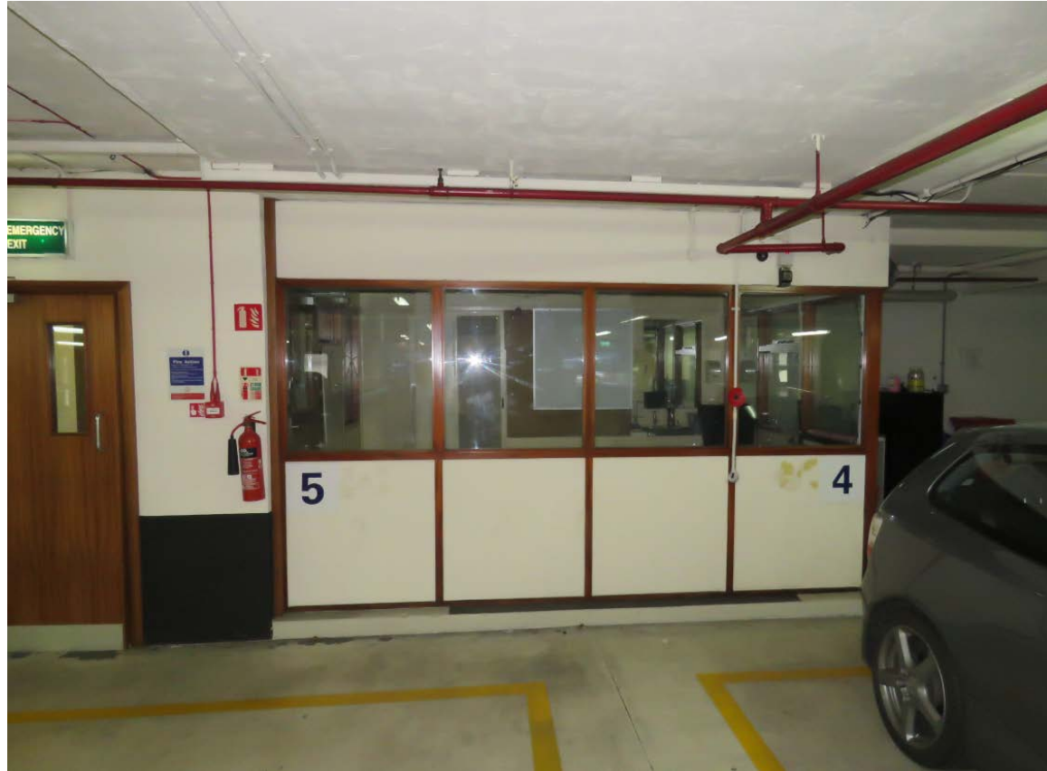
00m-08 Looking north towards the pedestrian entrance and the valet's office.
