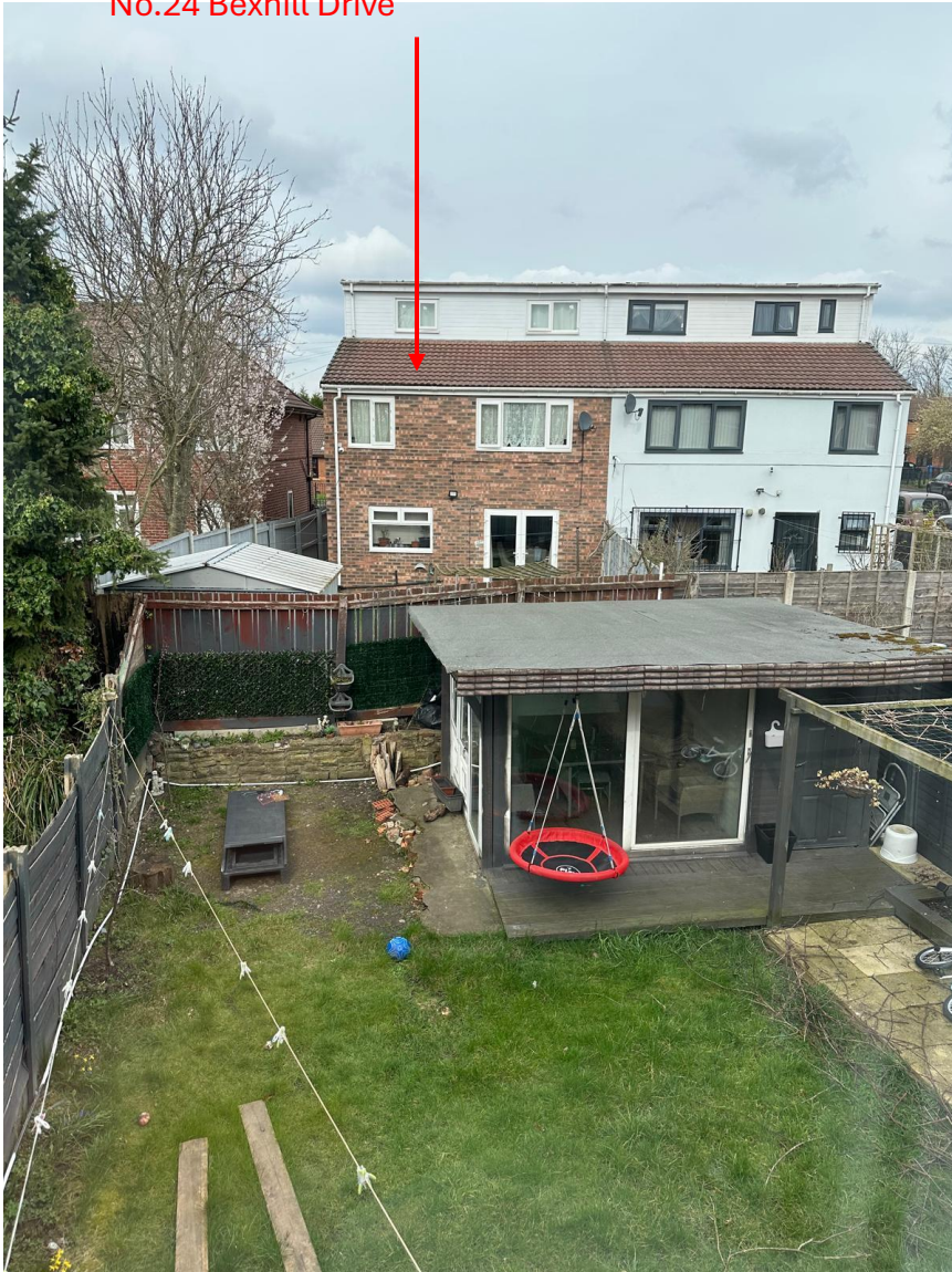
No.24 Bexhill Drive
