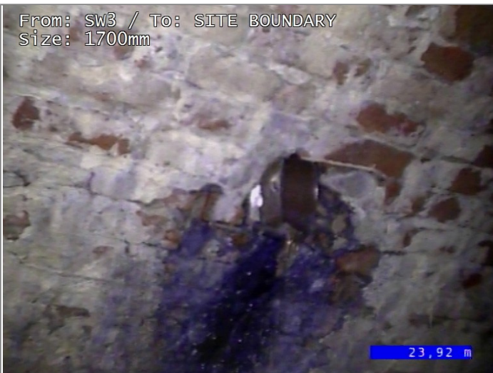
Connection other than junction at 9 o'clock, diameter 150mm
