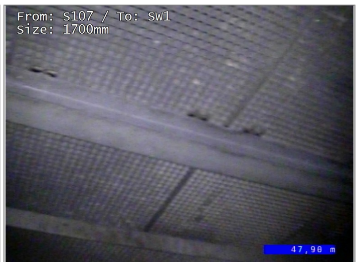
Finish node type, manhole, reference SW1
