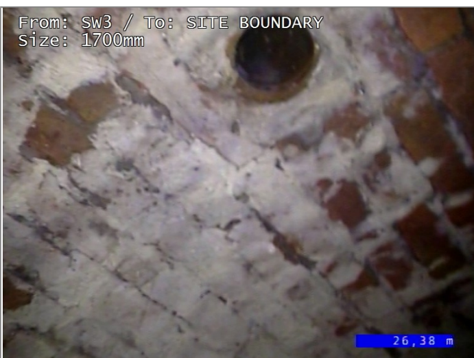
Connection other than junction at 12 o'clock, diameter 150mm
