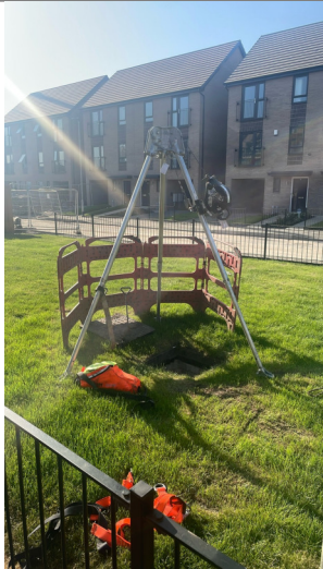
Other Site Photos: SW3 - All CCTV works carried out from this MH.
