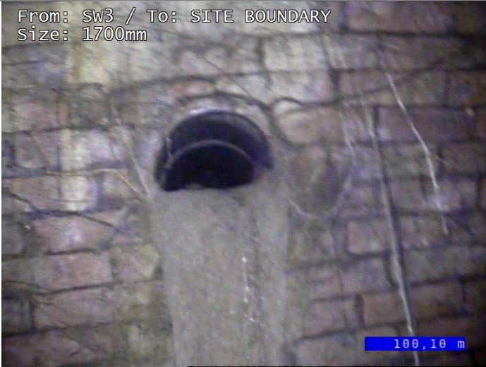
Junction, closed at 9 o'clock, diameter 225mm
