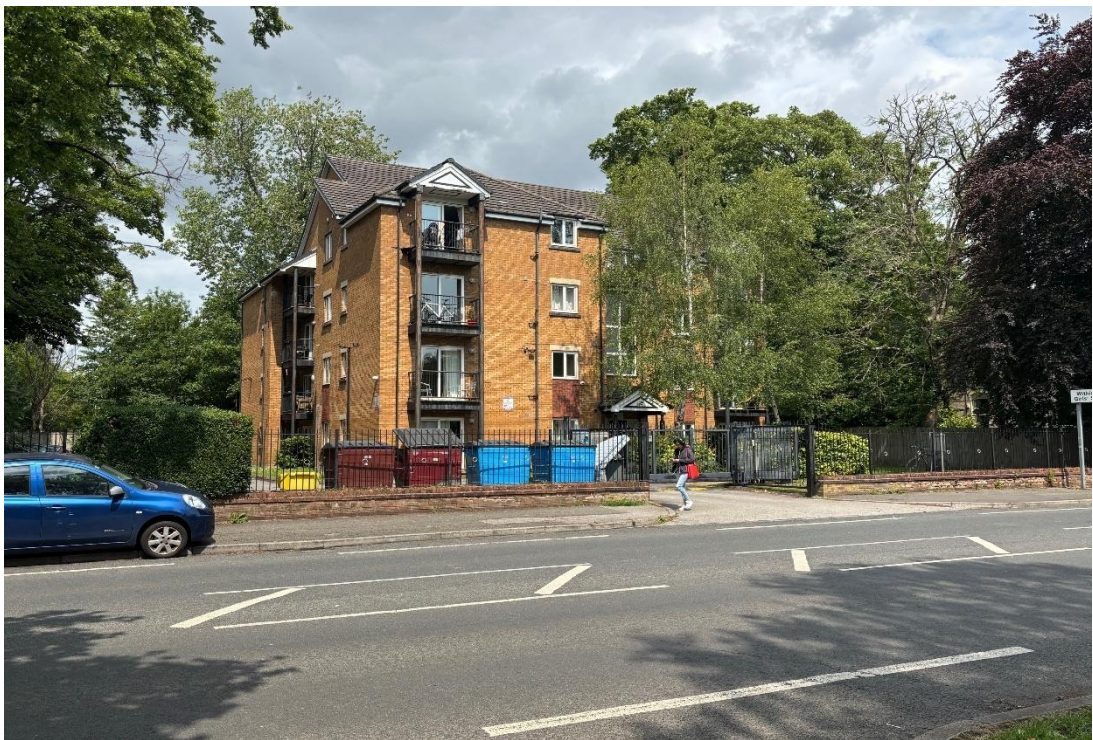
Figure 13 – Photograph of existing purpose built apartment block approximately 215 metres to east of site – June 2025
