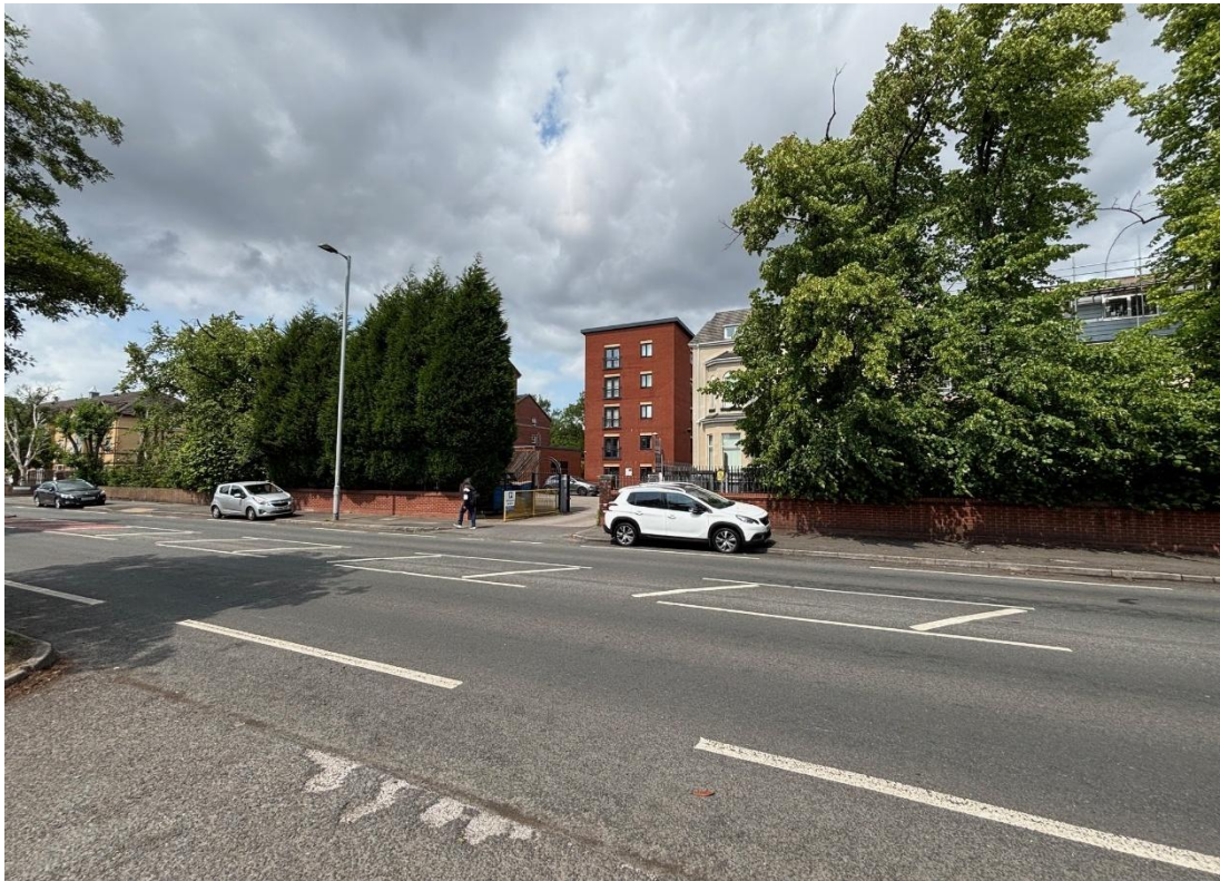
Figure 12 – Photograph of Wilbraham Court 2, approximately 150 metres east of the site – June 2025
