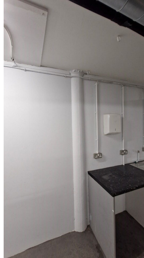
Plate 18: One of the cast iron columns encased a modern partition wall.
