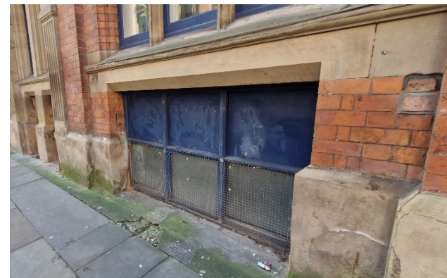
Plate 11: The basement windows to Princess Street.
