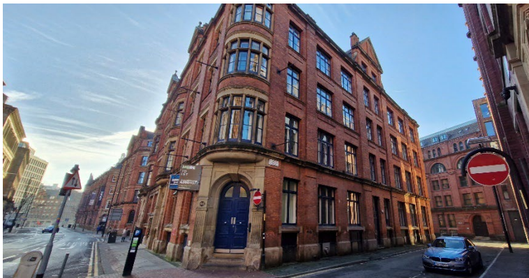
Plate 10: Transact House as seen from the north on Princess Street.
