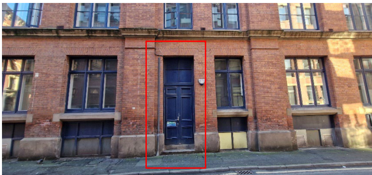
Plate 13: The modern door (no.1) providing access to the basement from Harter Street. This will be the customer entrance door.
