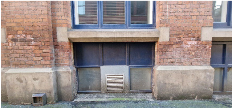
Plate 12: One of the basement windows to Harter Street, with ventilation grille inserted.
