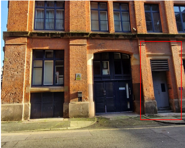
Plate 15: The secondary access/escape door (no. 2) from the basement on Harter Street.
