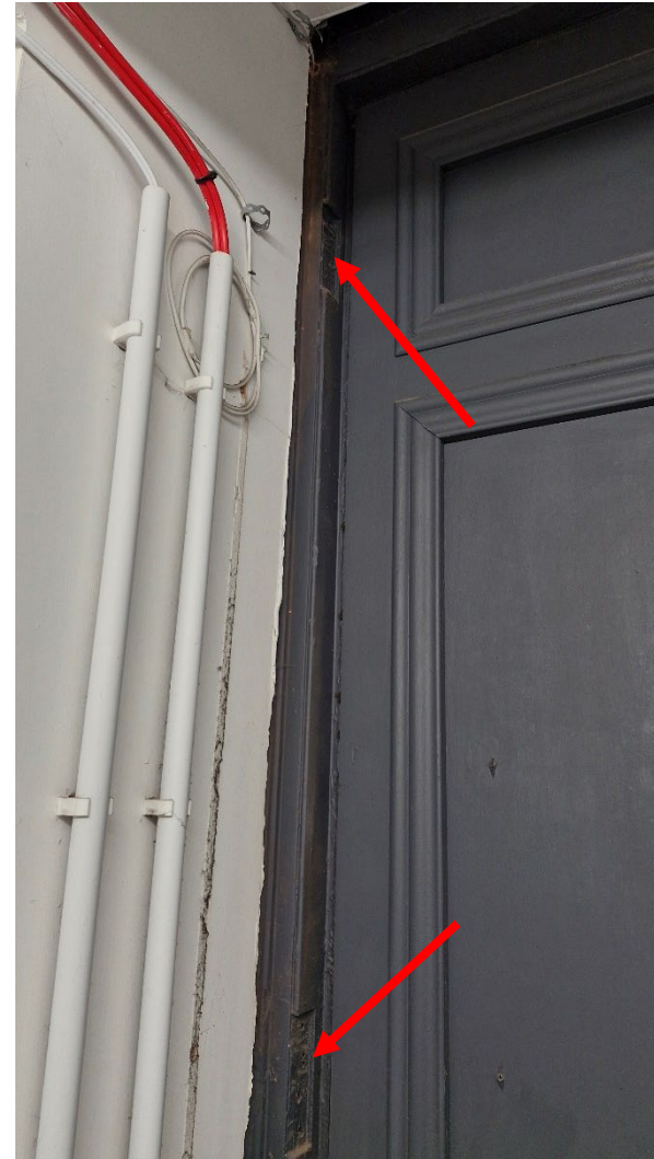
Plate 14: Evidence of earlier hinges to the doorframe to Harter Street.
