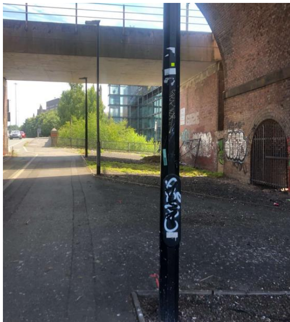
Figure 1 – Existing Egerton Street
