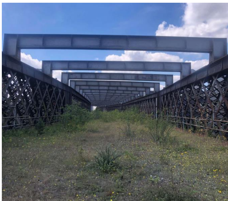
Figure 2 – Existing vacant viaduct (Phase 2)
