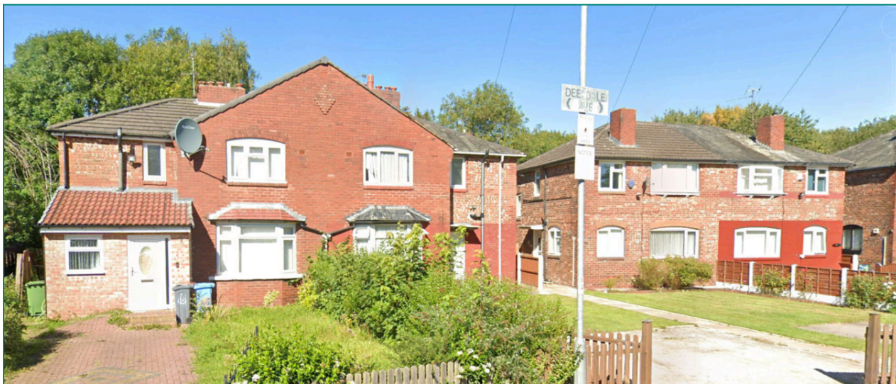
Figure 2: Properties 13-16 Deepdale Avenue
