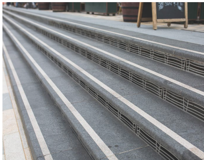
Integrated air vents; Battersea Power Station, London
