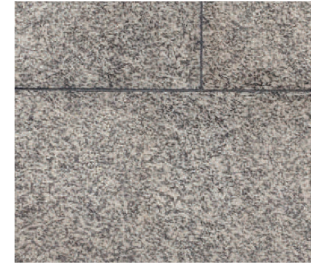
Existing stone cladding to facade
