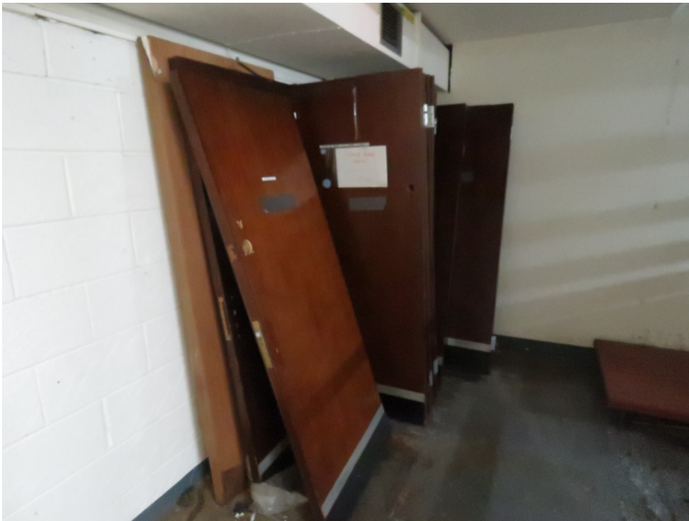
B2-13 View of original doors stored within basement.
