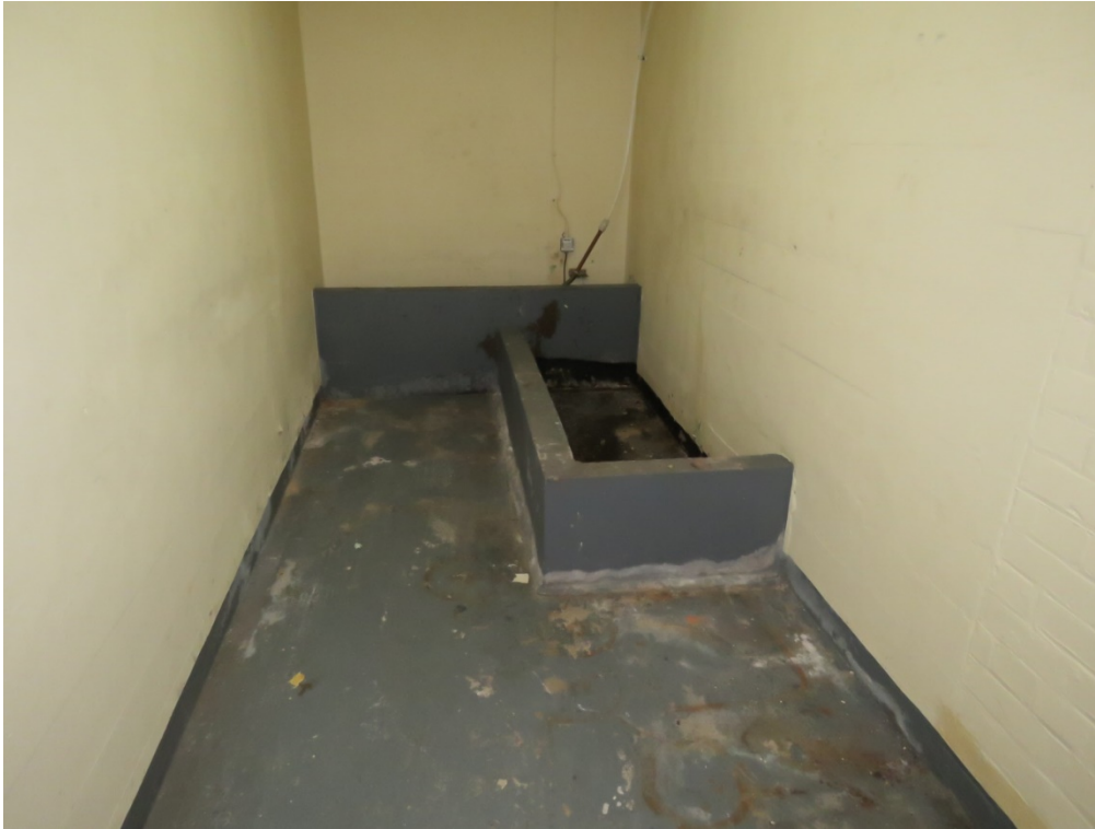
B2-06 View of one of the cleaning cupboards with concrete drain.
