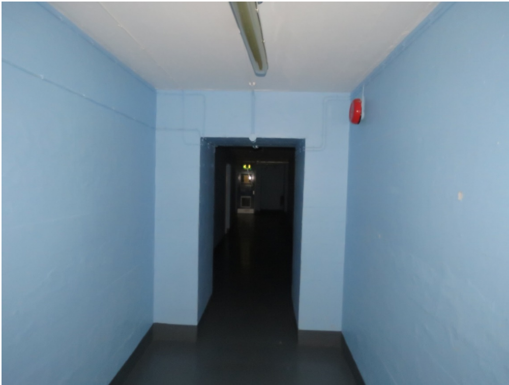
B2-01 View looking east along one of the primary corridors, note the painted shuttered concrete walls and ceiling.
