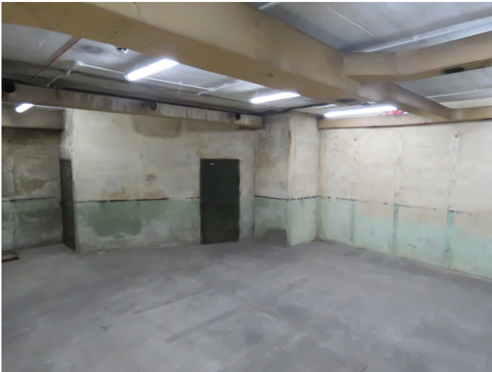
B2-11 View of room with original decoration, ventilation ductwork and riser.
