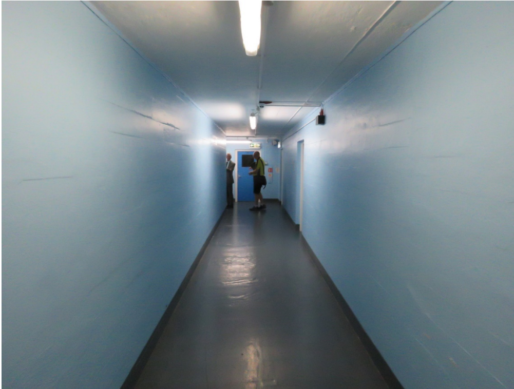
B2-02 View looking west along corridor.
