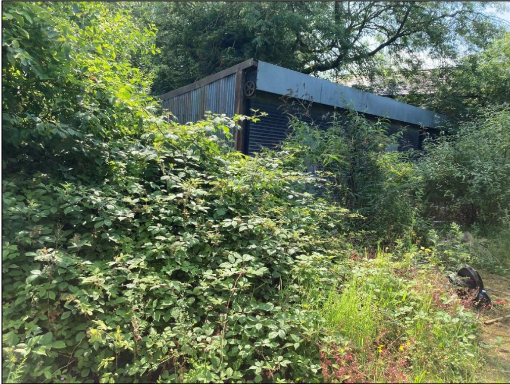
Plate 3 – Corrugated metal building occurring to the south of the site boundary
