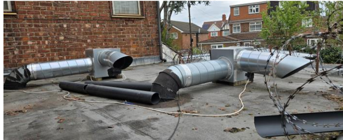
Figure 4 Flat roof to the rear where noise monitoring took place
