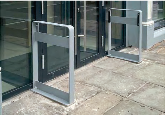
Existing door guarding
