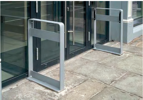
Existing door guarding
