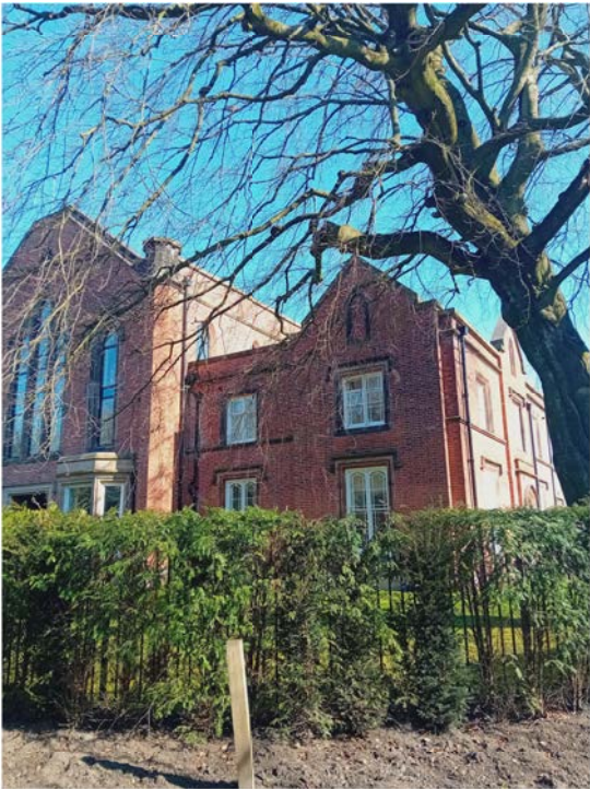
existing south-west elevation showing the roof terrace is not seen from the street.
