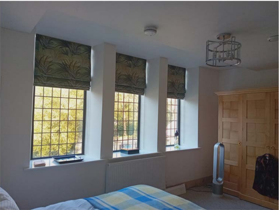
flat 9, first floor bedroom with no openable windows
