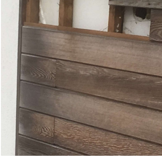
Existing timber cladding
