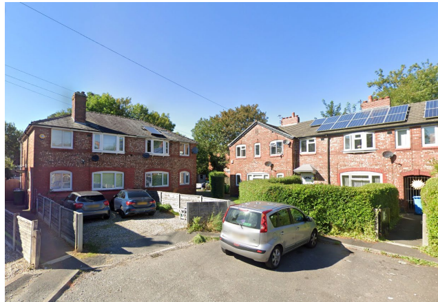
Residential Properties East Of The Proposed Site (Limehurst Ave)
