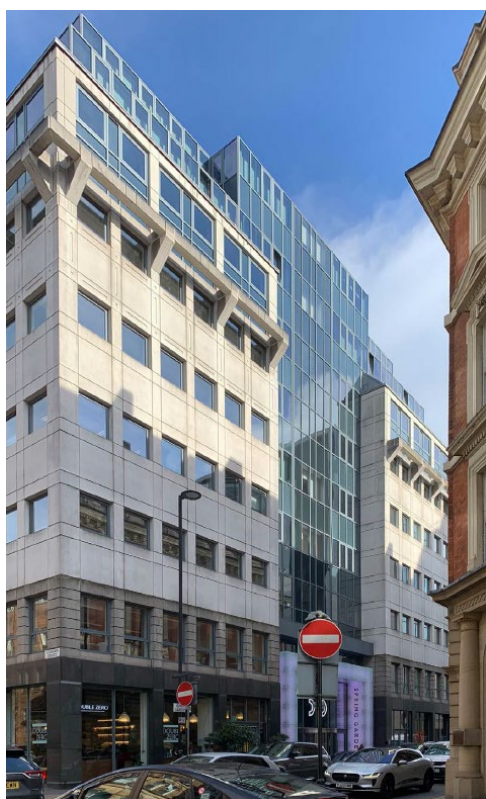
^ Figure 1: Existing building, viewed from Fountain Street
