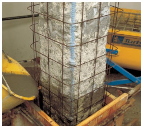
Pouring into a formwork
