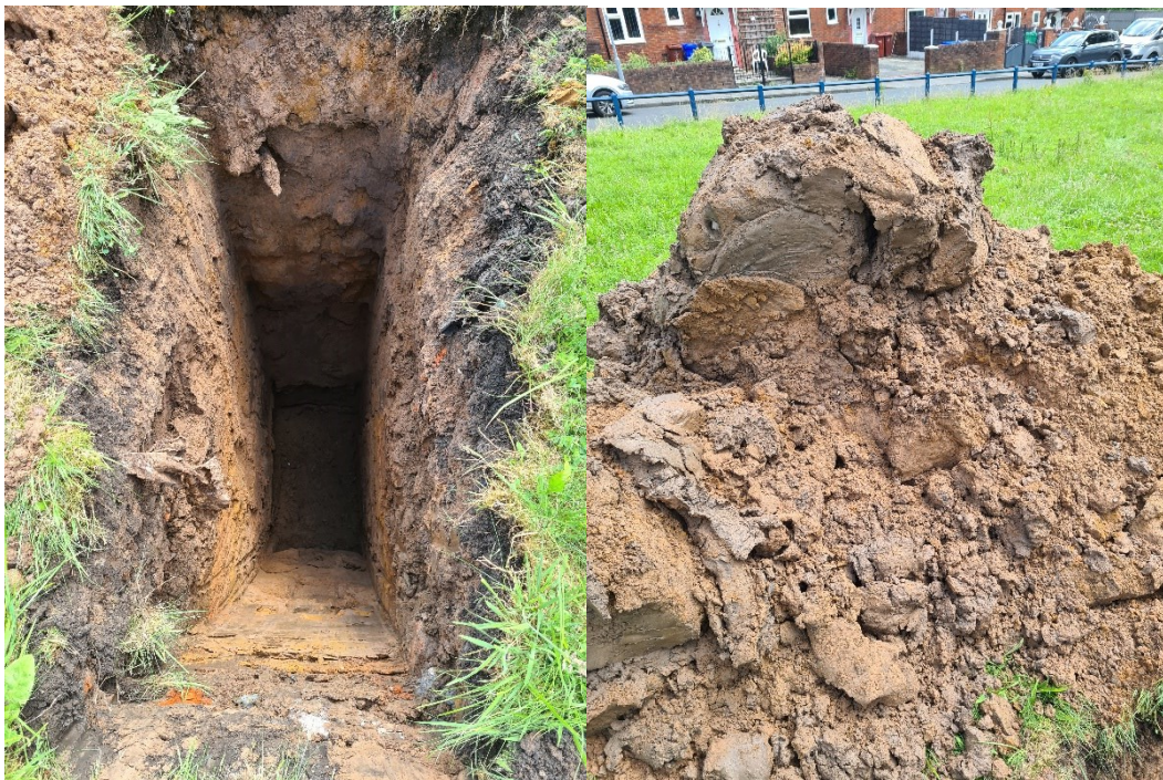
PLATE 8 TP107 EXCAVATION AND ARISING
