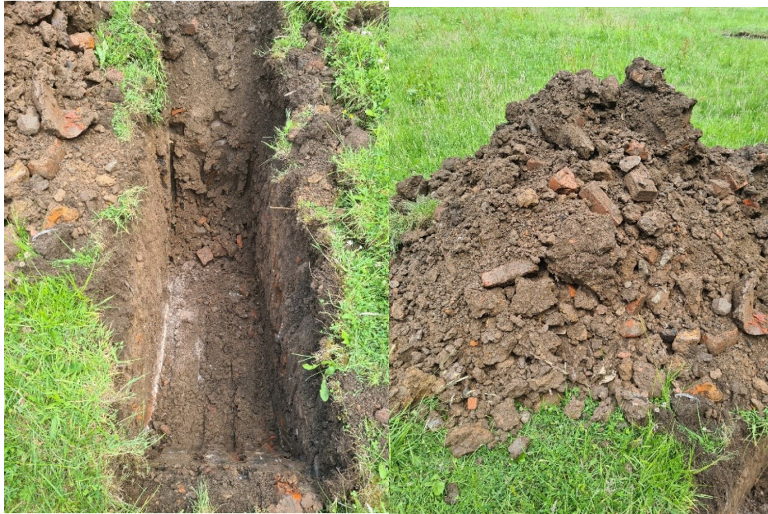
PLATE 9 TP109 EXCAVATION AND ARISINGS
