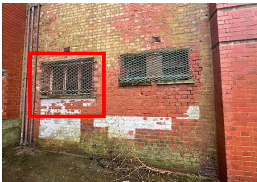
Figure 16: Existing windows in northern elevation.
