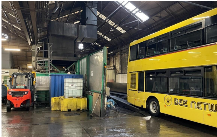
Figure 9: Existing bus chassis wash and wheel cleaning station
