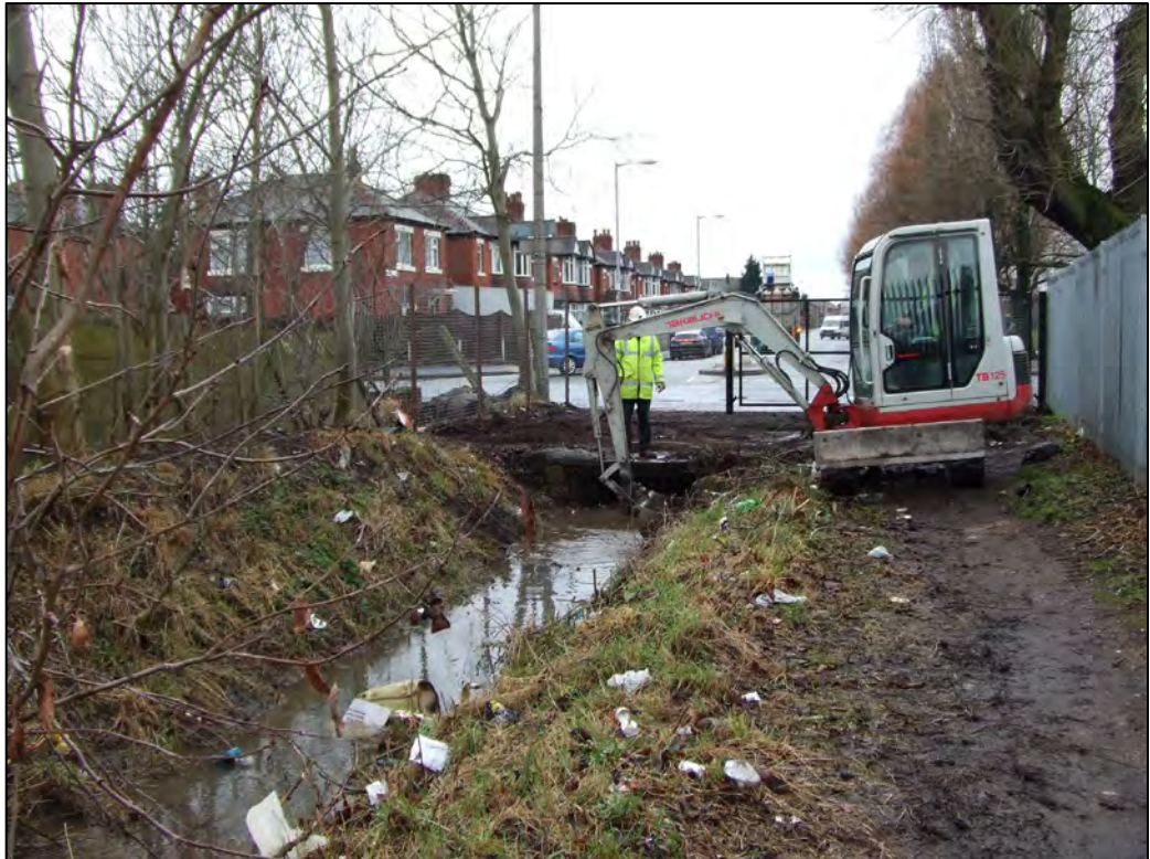
Figure 38: Clearing work at Nico Ditch at Gorton, 2008 during footpath building work.
