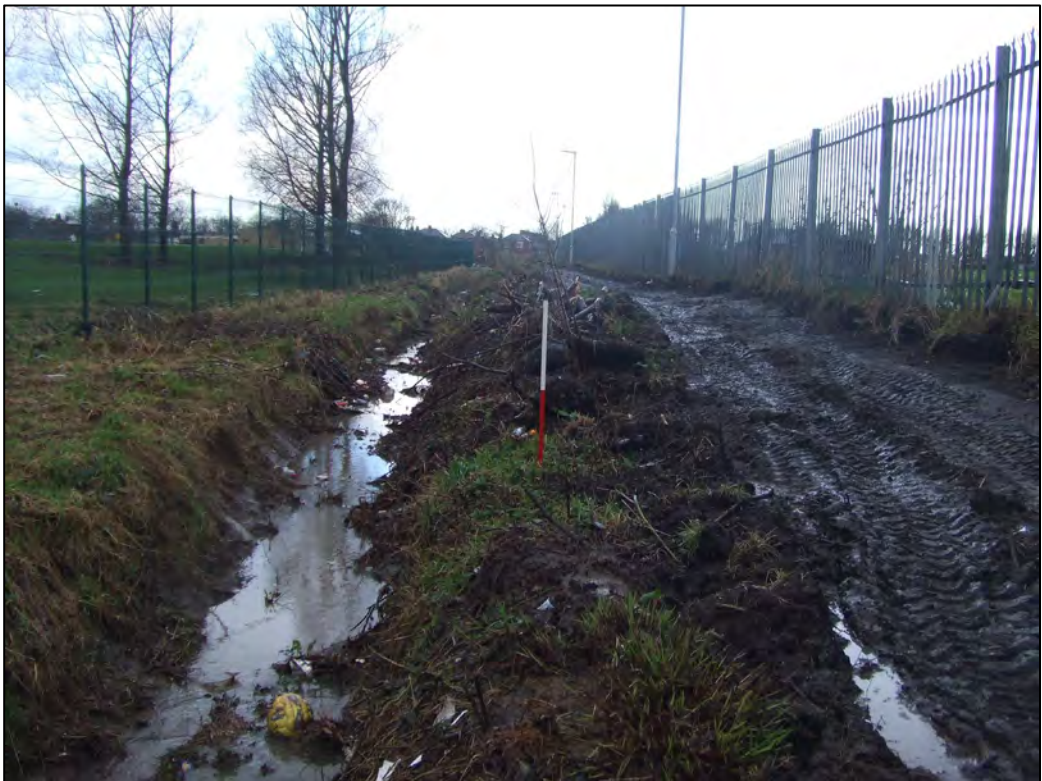
Figure 39: Recording work by UMAU during footpath building along Nico Ditch at Melland Playing Field, Gorton, 2008 during footpath building work.
