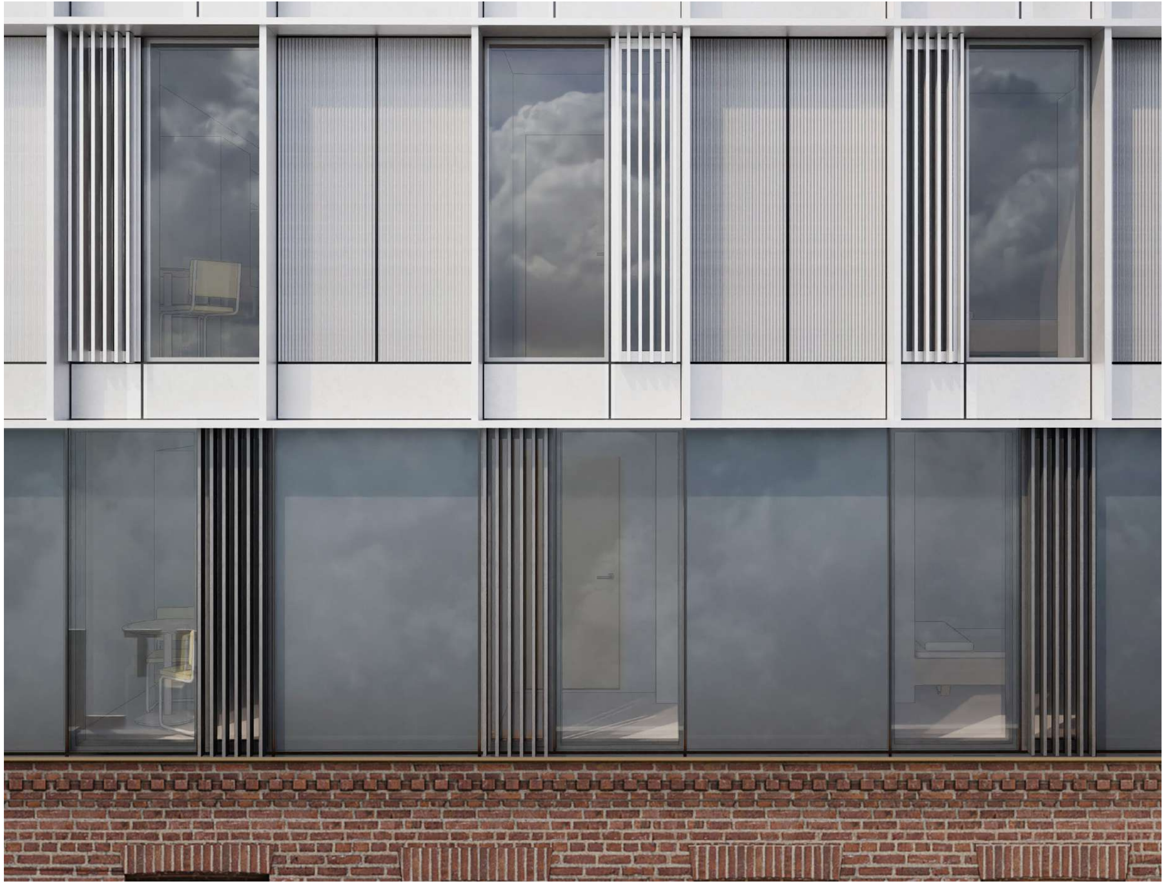
Visual extract illustrating the transition in materiality palette, from the brick podium, backsprayed 'neck' and Anolok 543 anodised aluminium tower.
