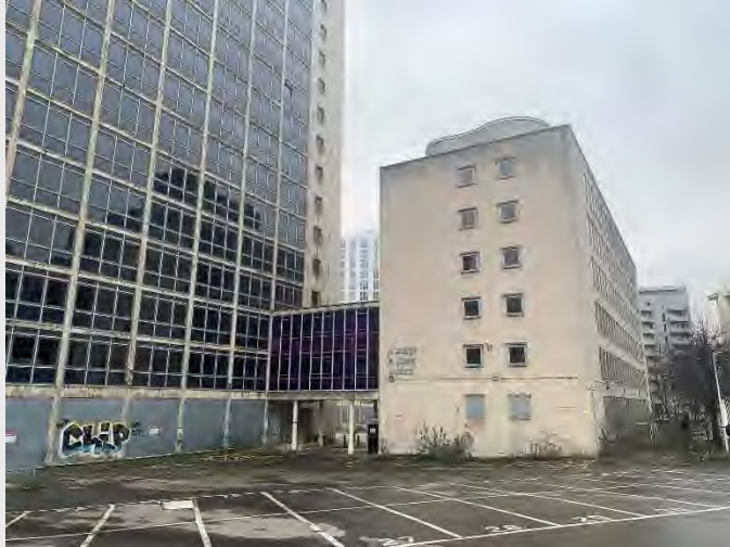
Photograph 1: Unused buildings and carpark
