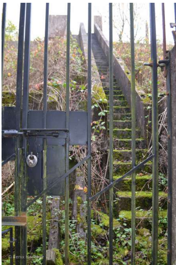
Plate 51: Sightline to the north towards steps and a ramp to the railway sidings.
