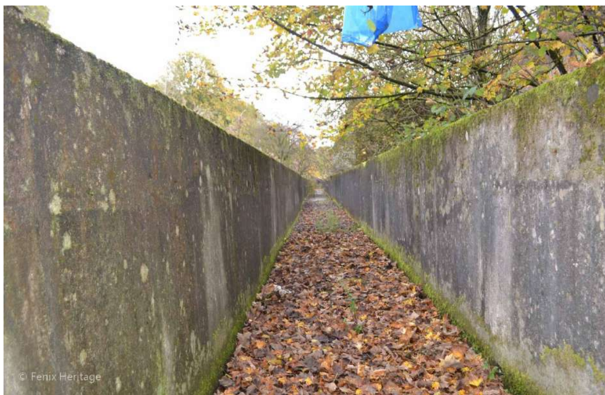
Plate 53: Sightline to the east along a walk-way on the north-facing elevation of the eastern bay, lairage, of the former Abattoir.
