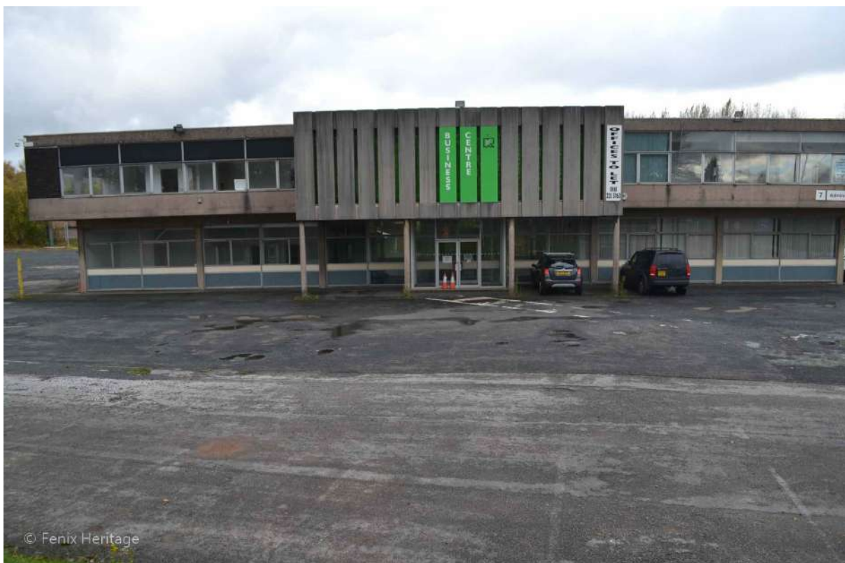
Plate 10: Sightline to the north to the south-facing elevation of the Administrative Block.
