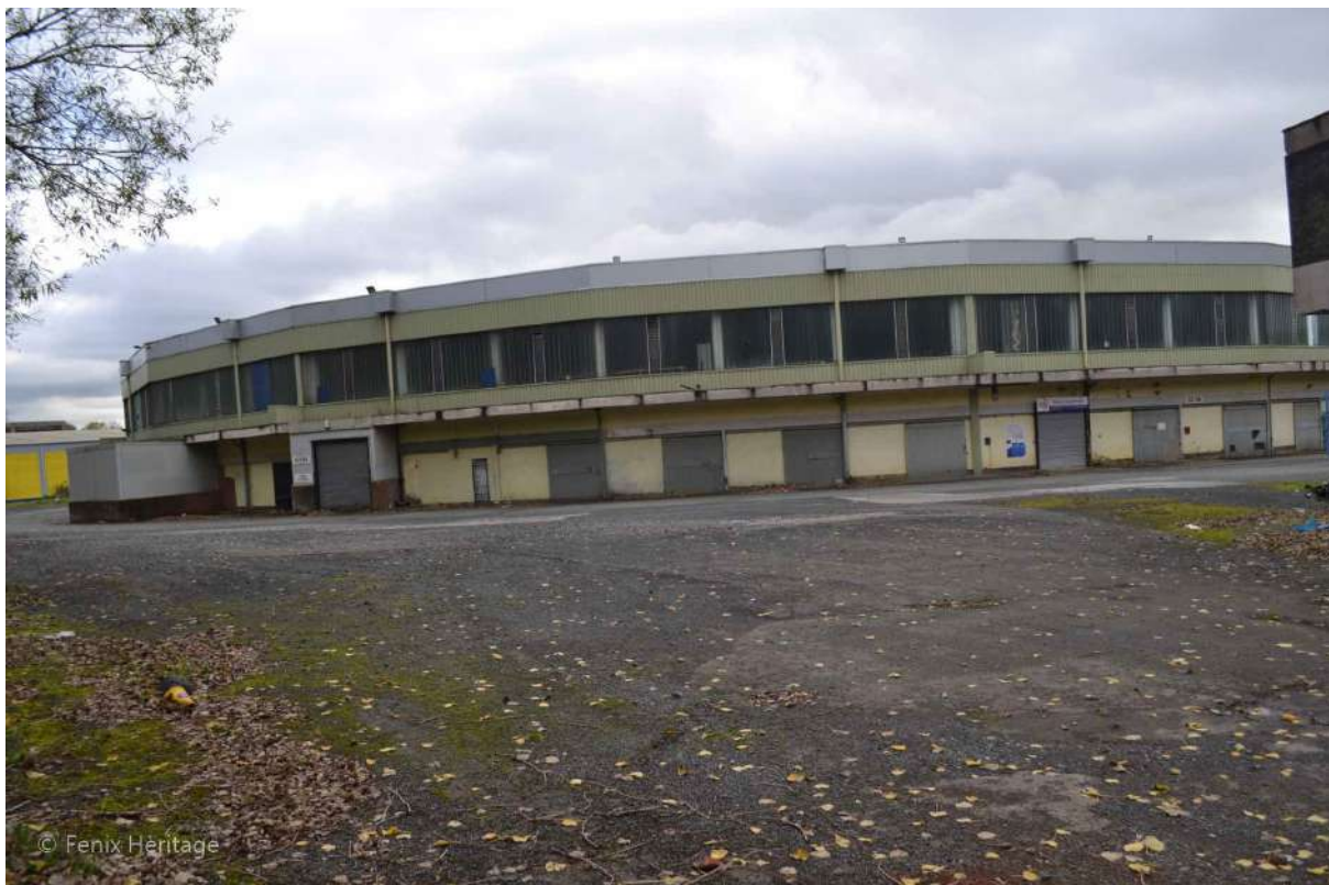
Plate 6: Sightline to the south-east towards the Meat Market. There was a high-level meat distribution system at first floor level over the traders' stalls at ground floor level.
