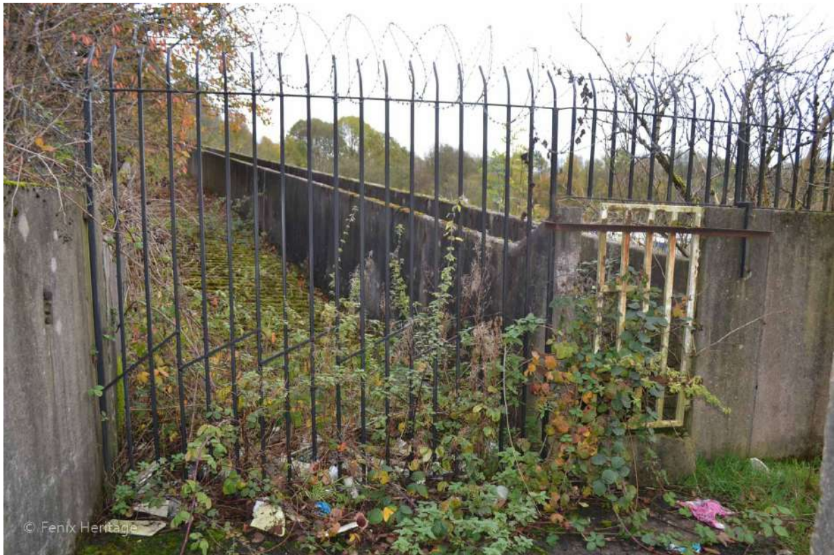
Plate 49: Sightline to east towards the terminal of the livestock ramp leading from the railway sidings.
