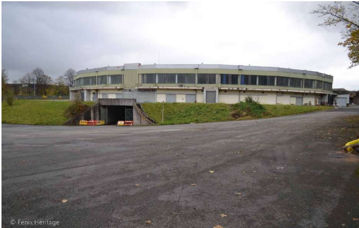
Plate 25: Sightline to the south-west across the hardstanding between the Abattoir and Meat Market. Subway to the Meat Market visible to left of centre. The gap in the fenestration at first floor level indicates the now blocked position of the terminal of the overbridge housing the elevated conveyor
