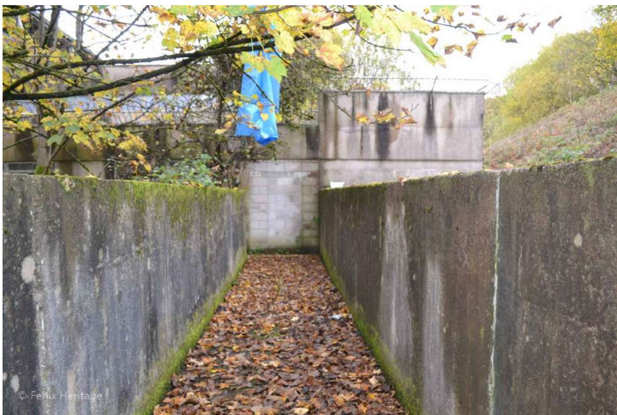
Plate 52: Sightline to the west towards a blocked doorway into the central bay of the former Abattoir.
