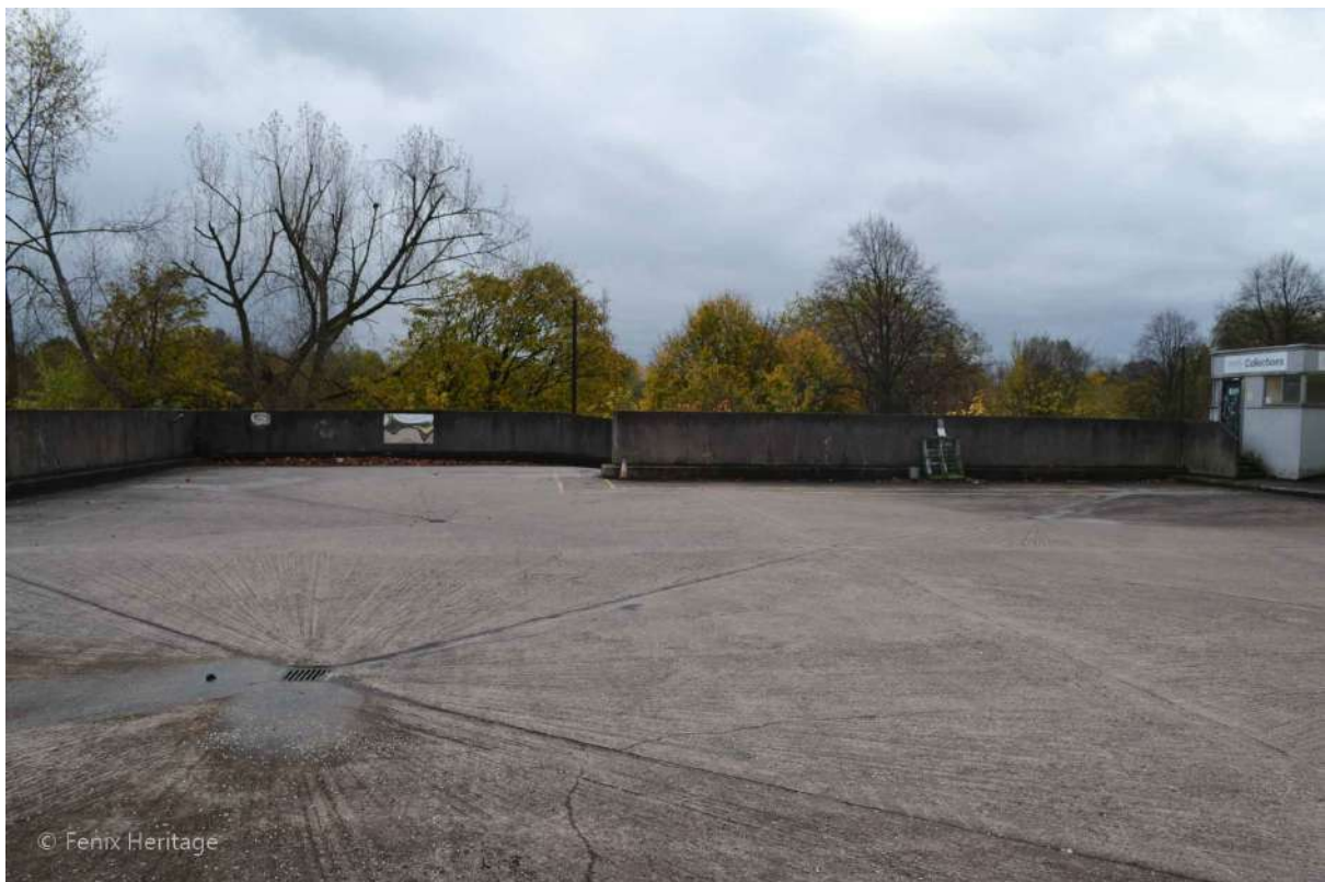
Plate 46: Sightline to the south across the vehicle deck of the eastern bay, lairage, of the former Abattoir.
