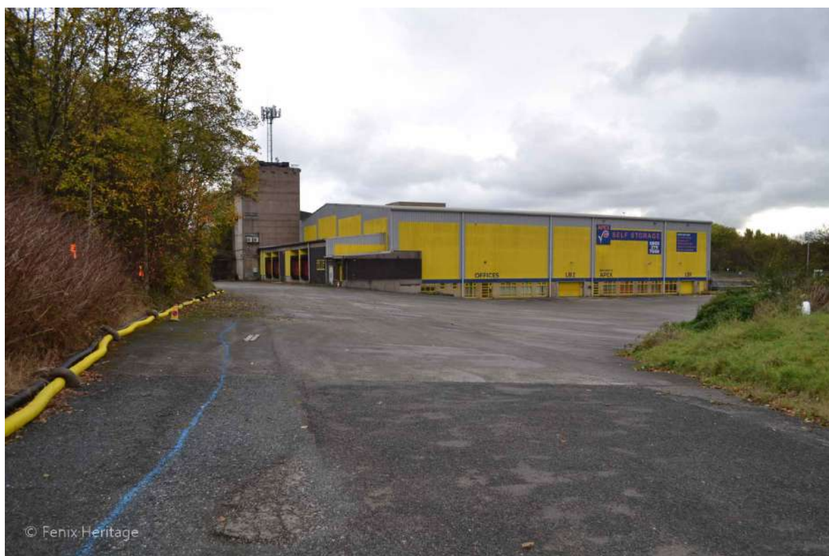
Plate 20: Sightline to the south-east towards the former cold store and chill rooms of the Abattoir. The tower was used for emergency slaughter.
