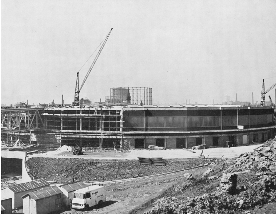
Meat Market during construction https://www.mainstreammodern.co.uk/city-abattoir-and-meat-market
