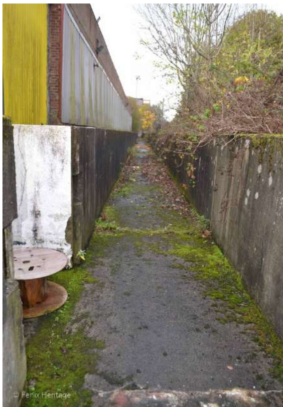
Plate 50: Sightline to the west along a walk-way on the north-facing elevation of the eastern bay, lairage, of the former Abattoir.
