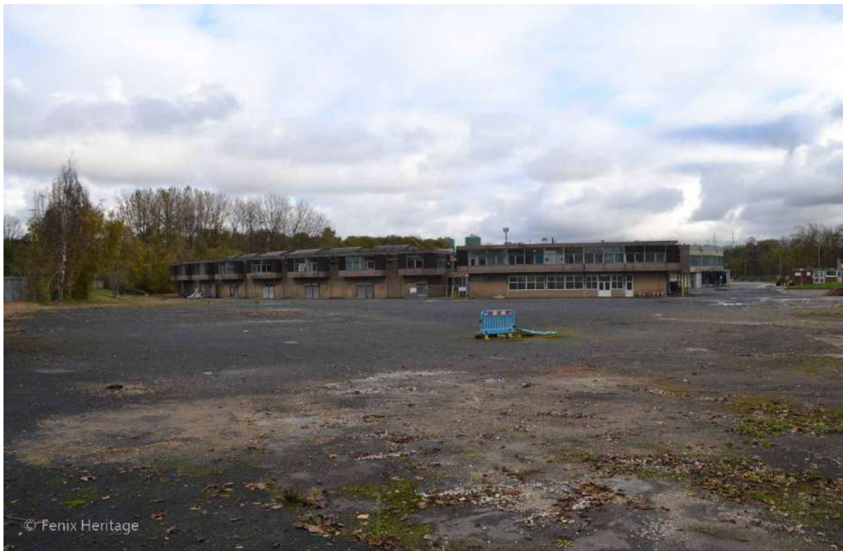
Plate 2: Sightline to the east towards the former Poultry Hall (at ground floor level) and Traders' offices (first floor) from the Site's south-western corner.
