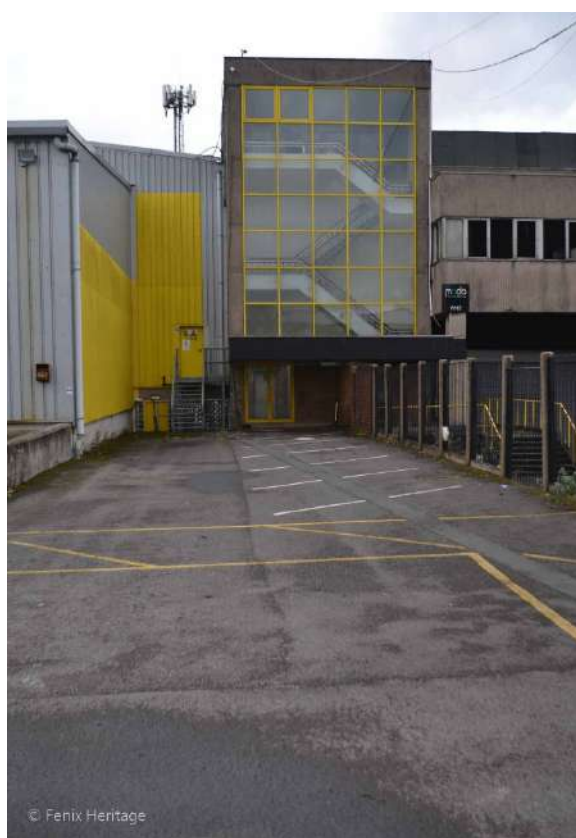
Plate 36: Sightline to the north highlighting the stairwell of the central bay (slaughter facility) of the former Abattoir.
