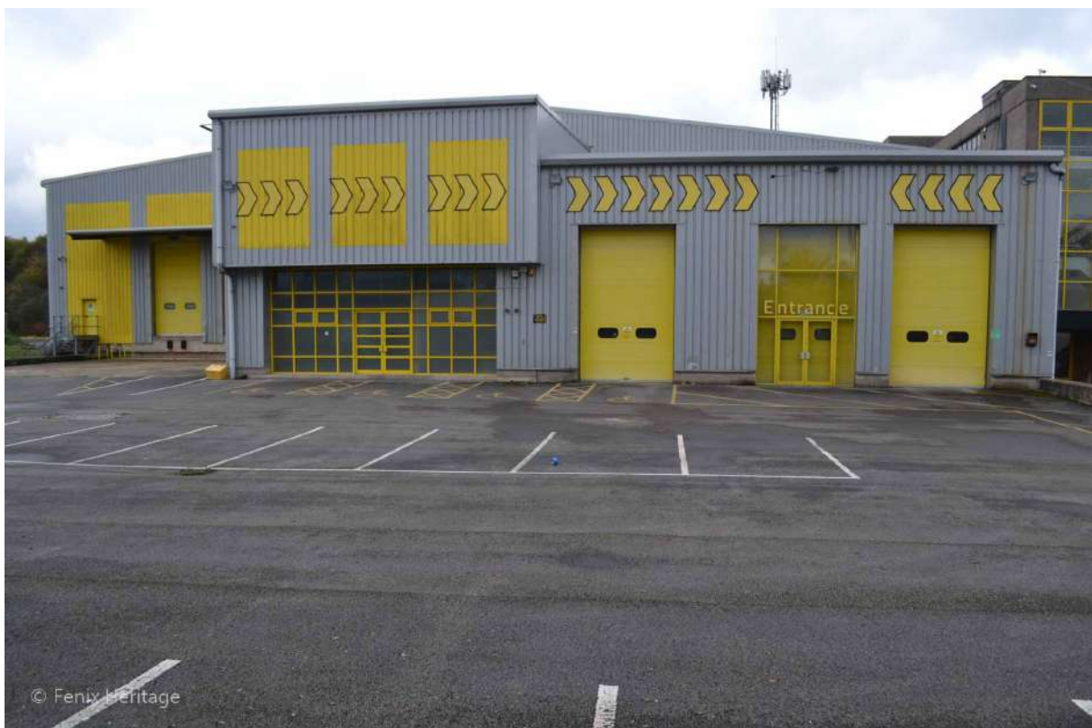
Plate 32: Sightline to the north to western bay of the rebuilt former cold store and chill rooms of the former Abattoir.
