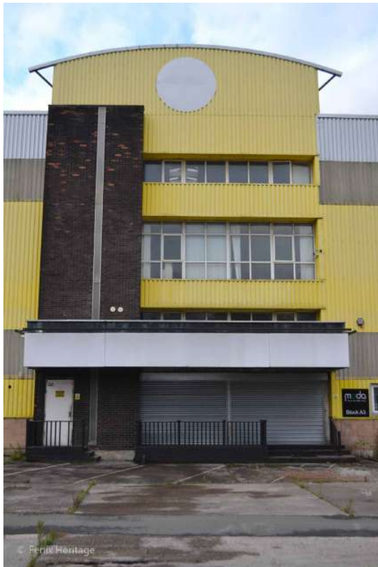
Plate 41: Sightline to the entrance to the eastern bay of the former lairage of the Abattoir.
