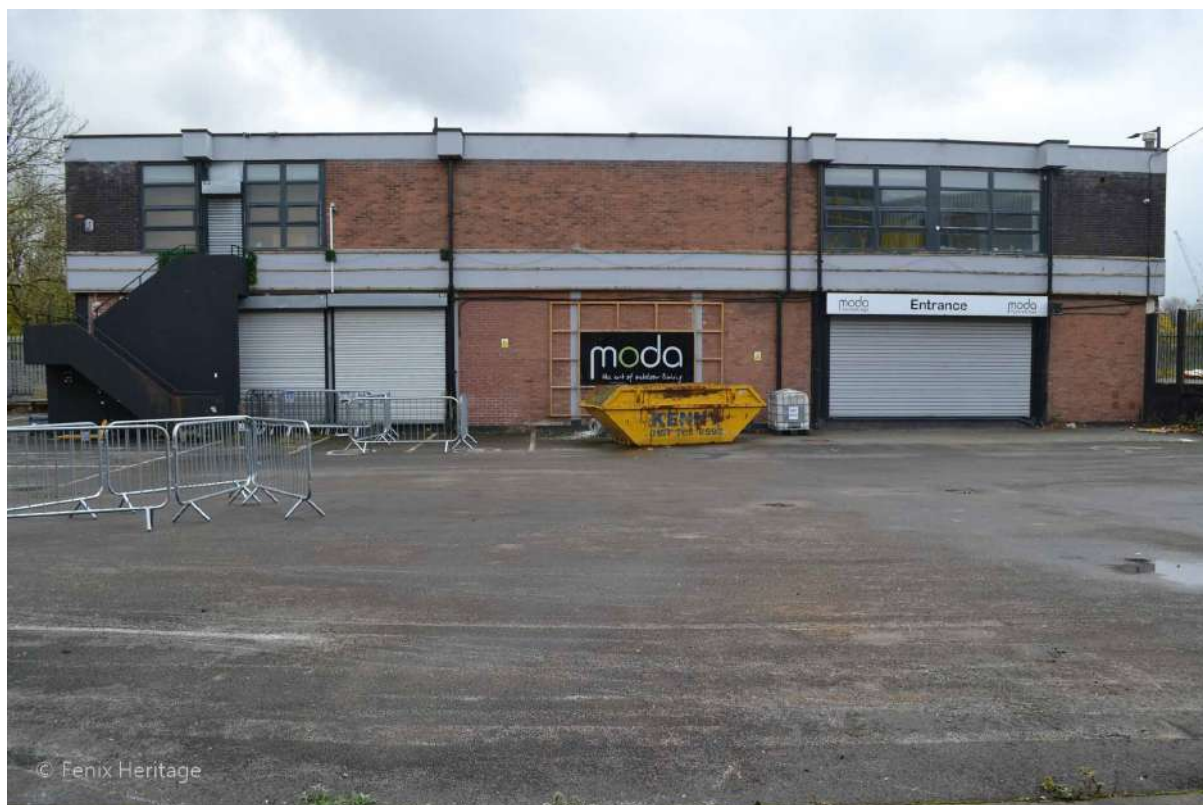
Plate 37: Sightline to the south to the north-facing elevation of the of the two-storey canteen block parallel to the Site's boundary with Riverpark Road.
