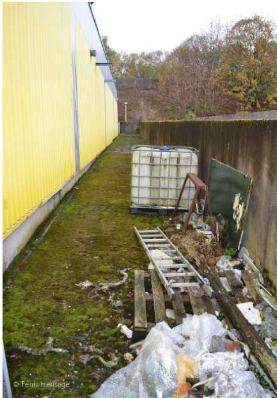
Plate 47: Sightline to the north along a walk-way on the east facing elevation of the eastern bay, lairage, of the former Abattoir.
