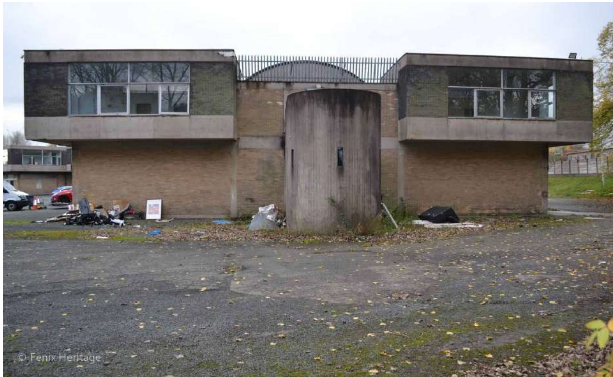
Plate 7: Sightline to the south to the rear (north-east facing) elevation of the former Poultry Hall (at ground floor level) and Traders' offices (first floor)
