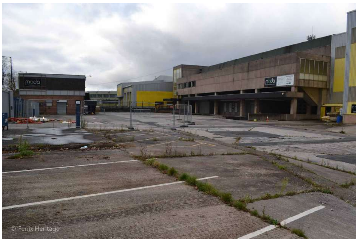
Plate 40: Sightline to the north-west towards the central and western bay of the former Abattoir.
