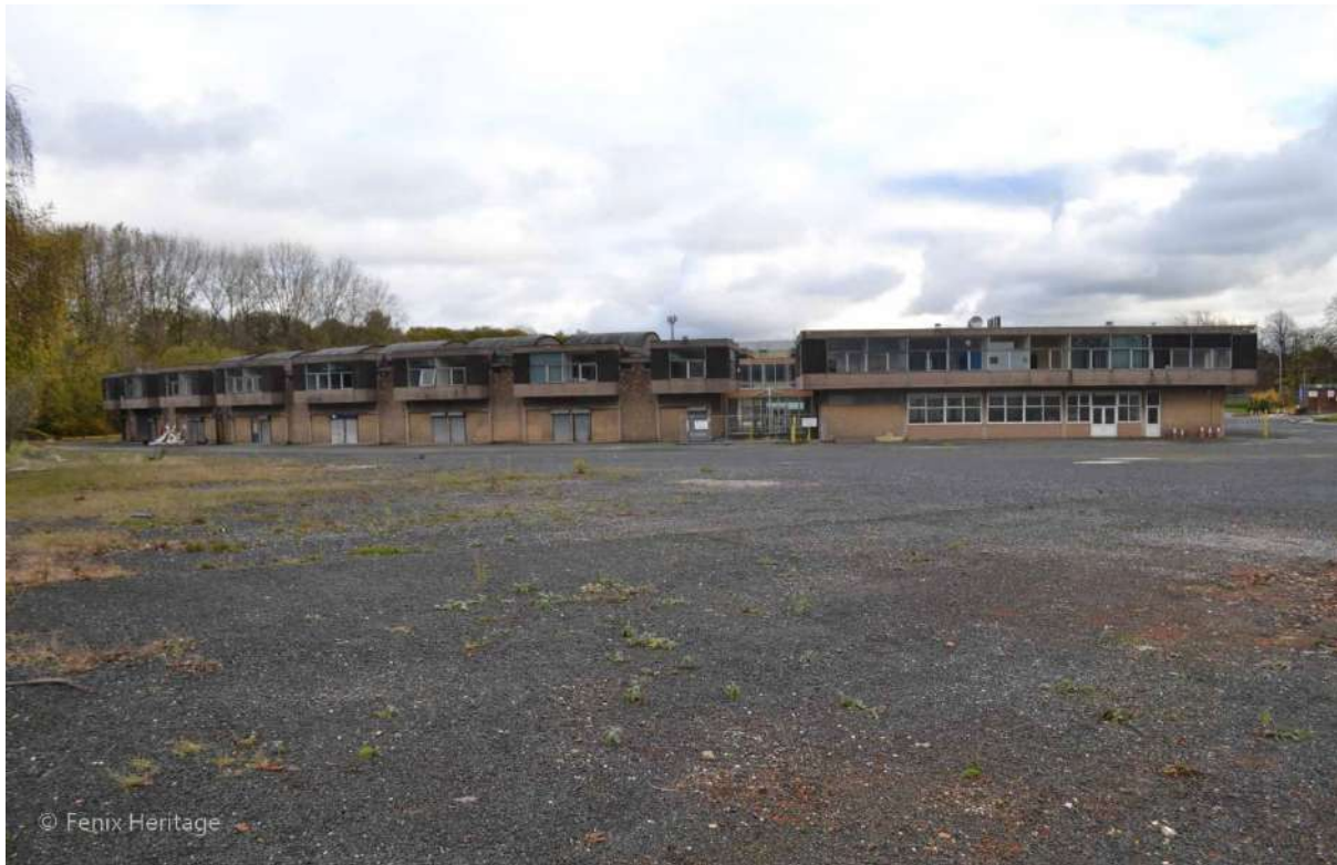
Plate 3: Sightline to the east towards the former Poultry Hall (at ground floor level) and the cantilevered Traders' offices (first floor). The open space in front of the right-hand end of the structure may contain archaeological remains of a Hoffmann Kiln which served the Jacksons' Brick Works.
