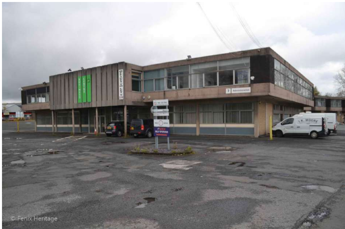
Plate 13: Sightline to the north-west to the south-facing elevation of the Administrative Block.
