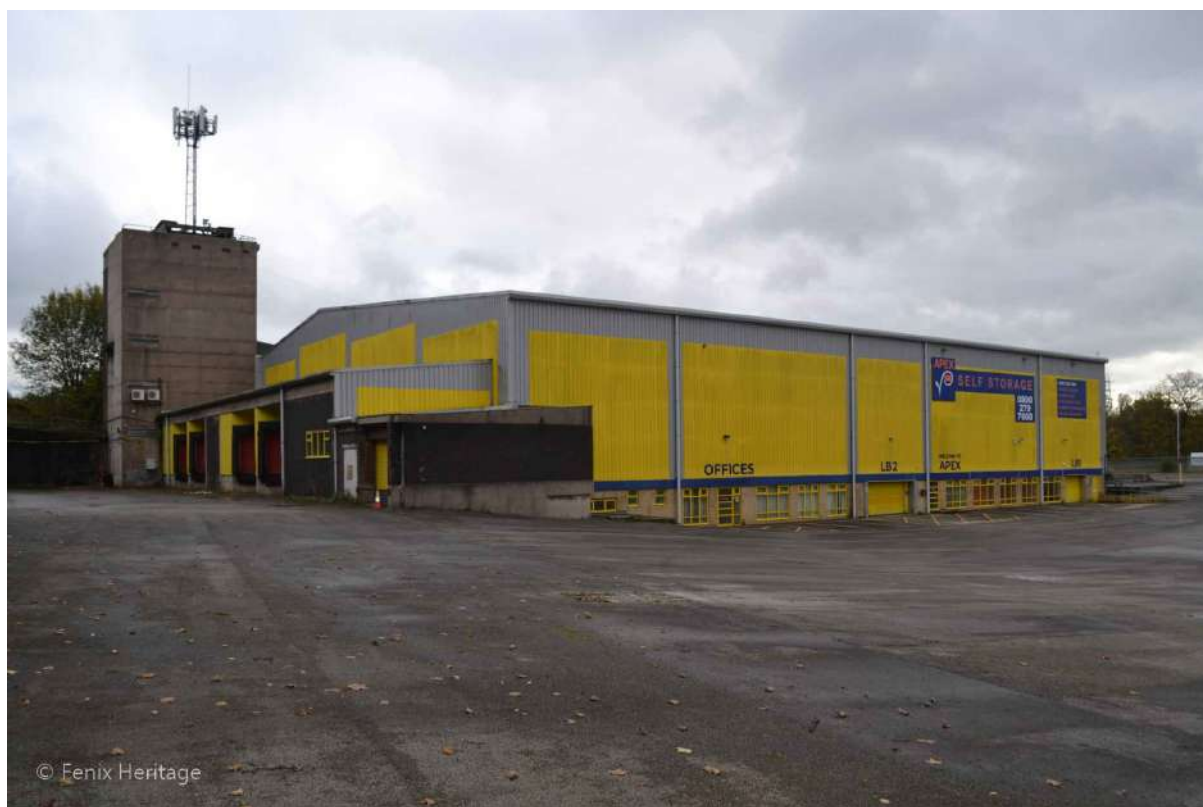
Plate 24: Sightline to the south-east towards the cold store and chill rooms of the Abattoir.
