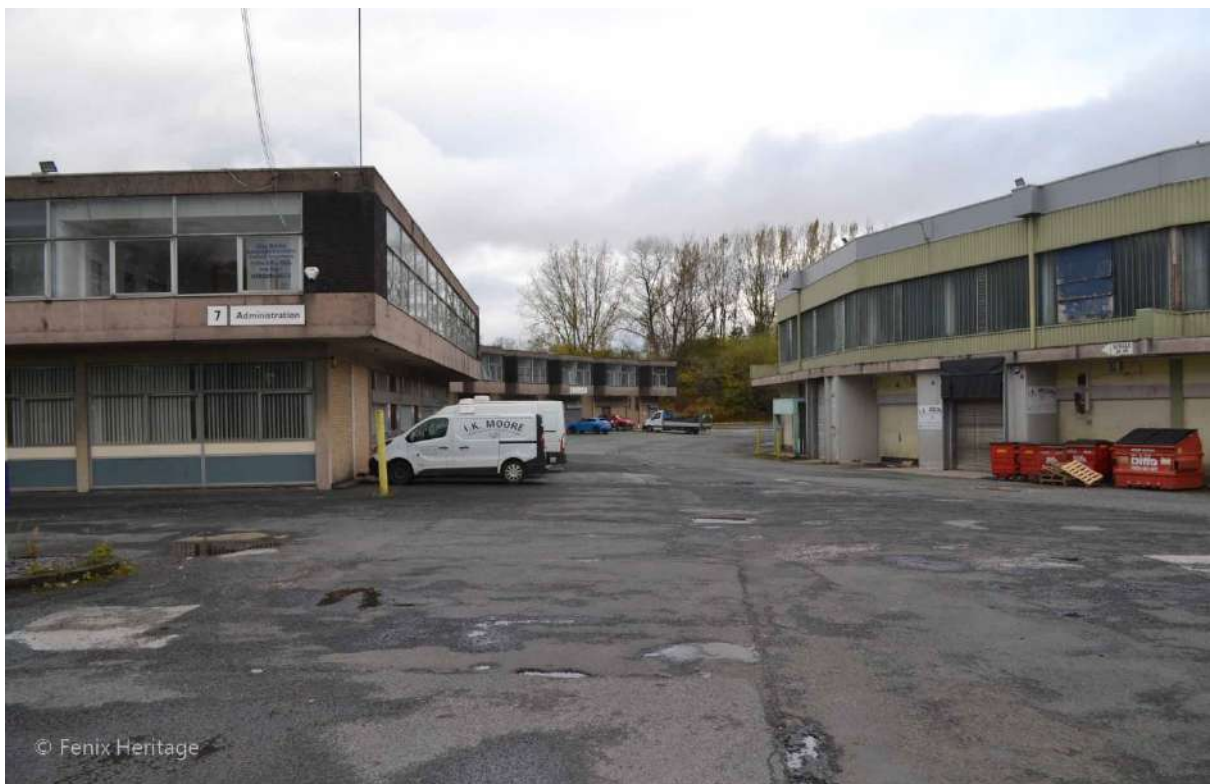
Plate 12: Sightline to the north along the access way between the Administrative Block (left) and the Meat Market (right). This is an area in which archaeological remains of a Hoffmann Kiln for the Jacksons' Brick Works may survive.
