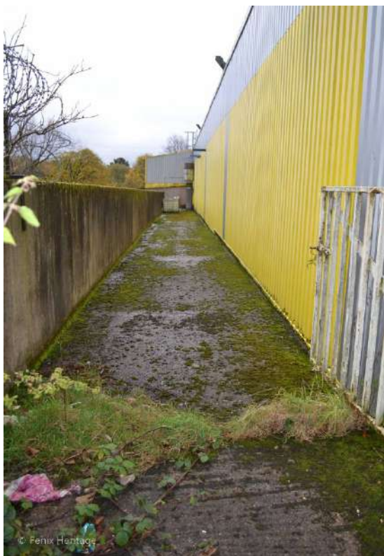
Plate 48: Sightline to the south along a walk-way on the east facing elevation of the eastern bay, lairage, of the former Abattoir.
