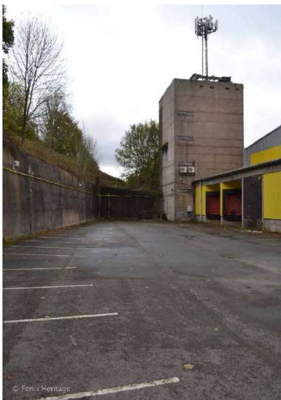
Plate 22: Sightline to the east along the yard between the rear of the cold store and chill rooms and the retaining wall to the railway embankment.
