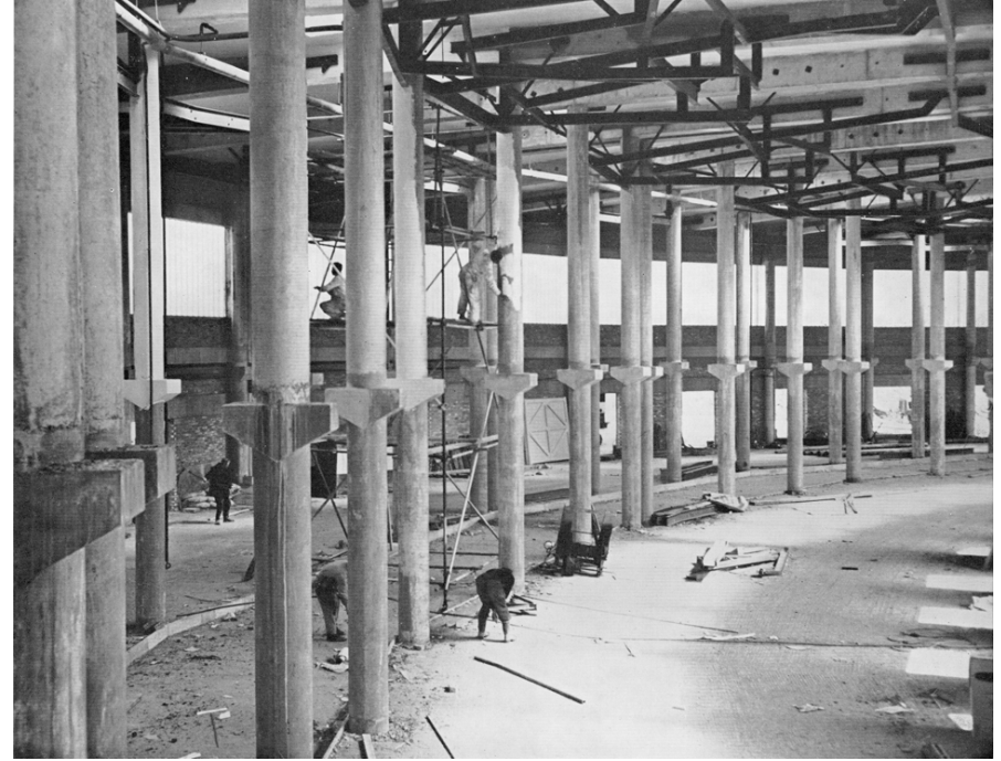
Meat Market during construction https://www.mainstreammodern.co.uk/city-abattoir-and-meat-market
