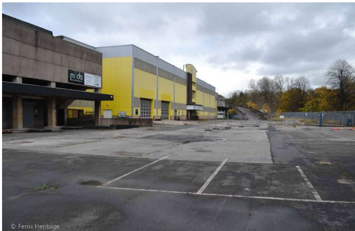
Plate 38: Sightline to the east towards the eastern bay (lairage) of the former Abattoir. It was re-clad c. 2002 using yellow corrugated panels.
