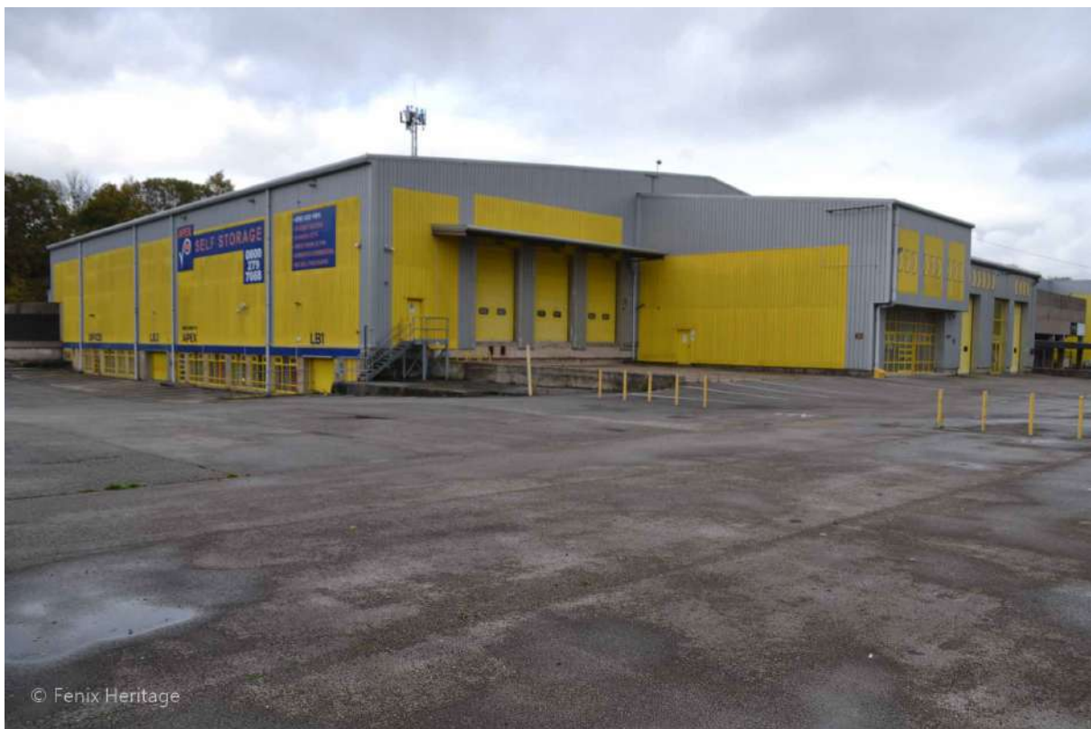
Plate 28: Sightline to the north-east towards the former cold store and chill rooms of the Abattoir.
