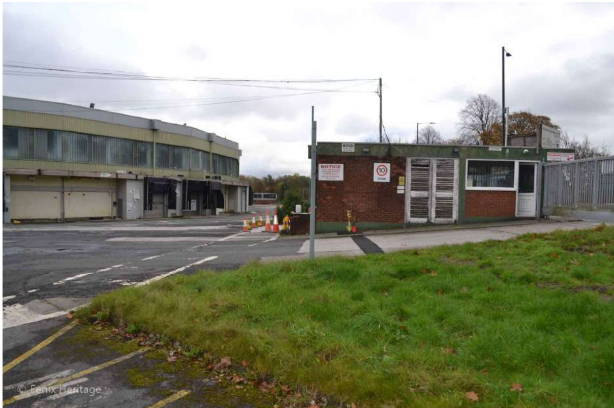
Plate 9: Sightline to the east towards the security lodge and vehicle entrance to the Site.
