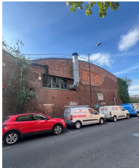
Brick frontage fronting Ducie Street
