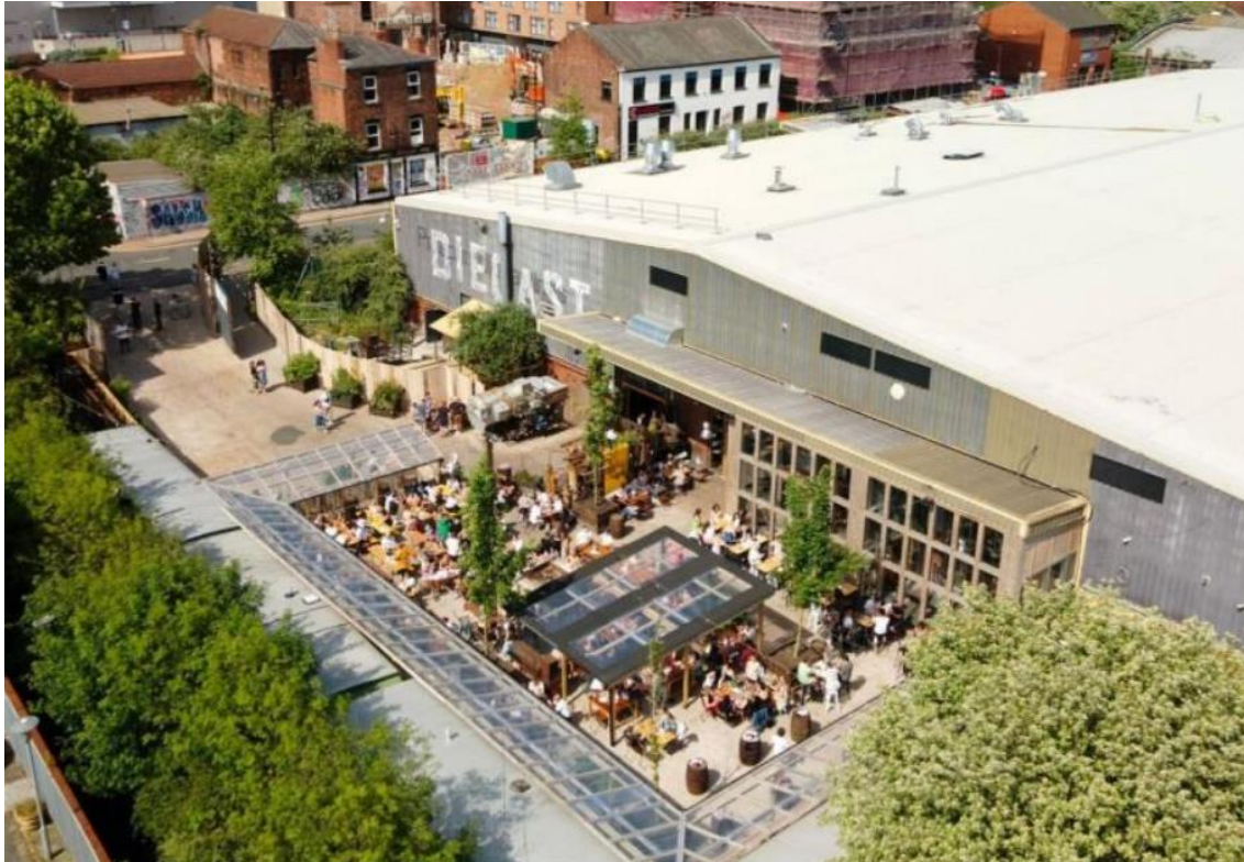
Aerial photo of building and outdoor seating area
