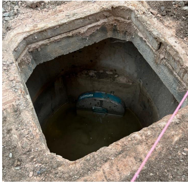
Photograph showing the construction of the private flow control chamber S11 have been constructed in accordance with DCG guidance and Hydro International specialist design drawings.
