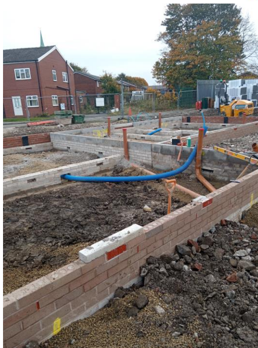
Photographs showing the construction of the internal foul drainage pop ups beneath the finished slab level, with direct connections to the external polypropylene inspection chambers.
