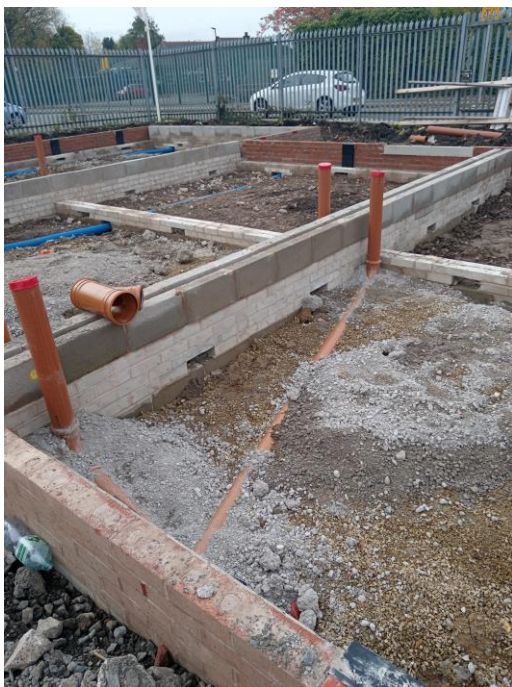
Photographs showing the construction of the internal foul drainage pop ups beneath the finished slab level, with direct connections to the external polypropylene inspection chambers.
