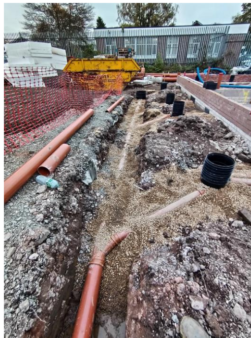
Photographs showing the construction of the main below ground drainage systems on site, pipes are laid with suitable bedding, in approved materials and with correct junctions and connections from plot drainage.
