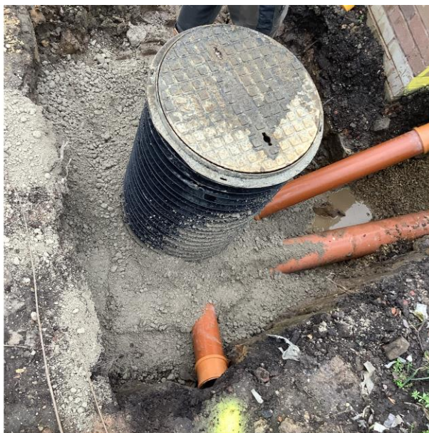
Photographs showing the construction of plot FW polypropylene inspection chambers outside each property in accordance with CDP drawing 21.B.13126-200 Engineering Appraisal and Building Regulations Document H.
