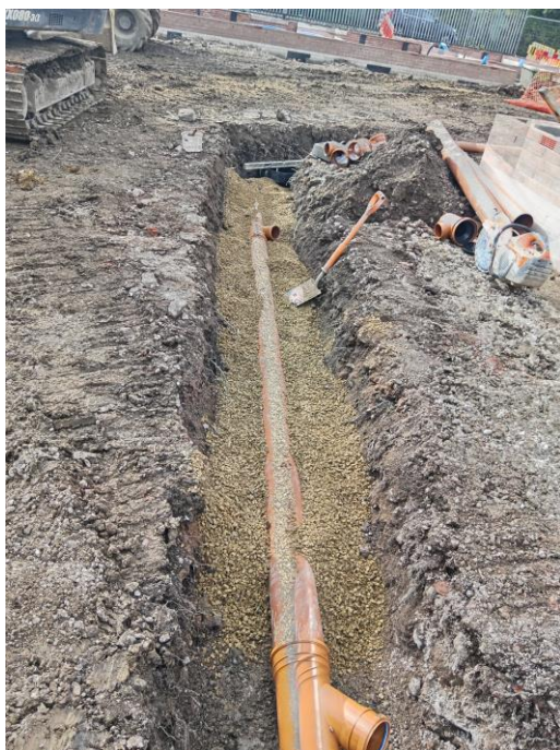
Photographs showing the construction of the main below ground drainage systems on site, pipes are laid with suitable bedding, in approved materials and with correct junctions and connections from plot drainage.
